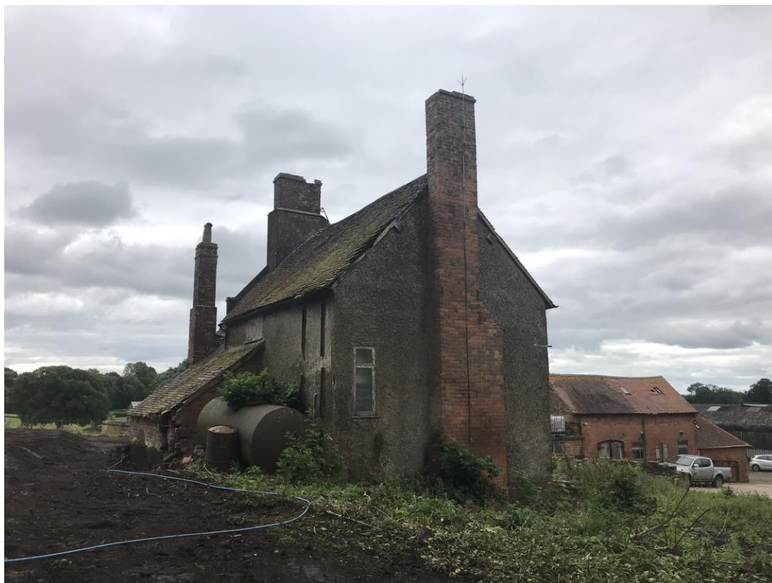
PHOTO 5 – FARMHOUSE FROM NORTH-WEST
