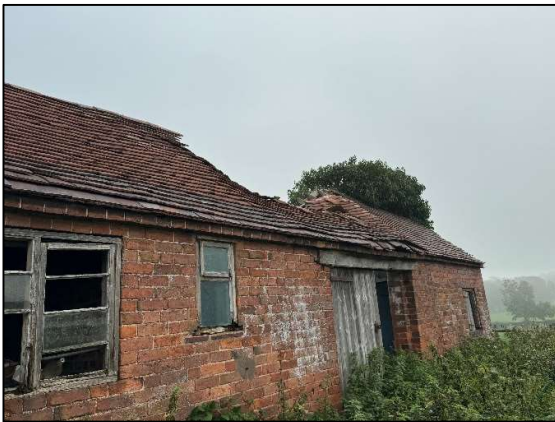
Photo 6: South Elevation of Adjoining Barn
