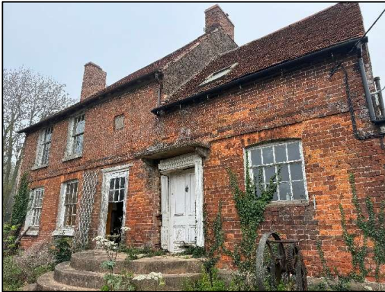
Photo 1: South Elevation of Farmhouse
