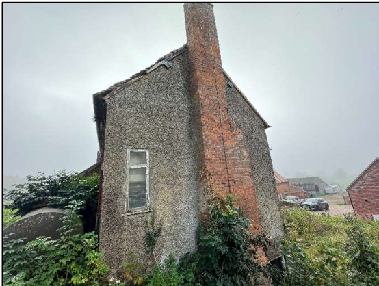
Photo 2: West Elevation of Farmhouse
