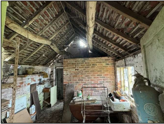
Photo 29: Internal View of Adjoining Barn (western end)
