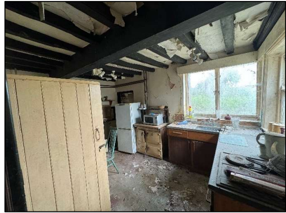
Photo 32: Internal View of Kitchen
