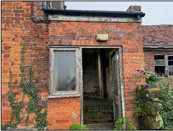
Photo 5: South Elevation of Single Storey Link Building
