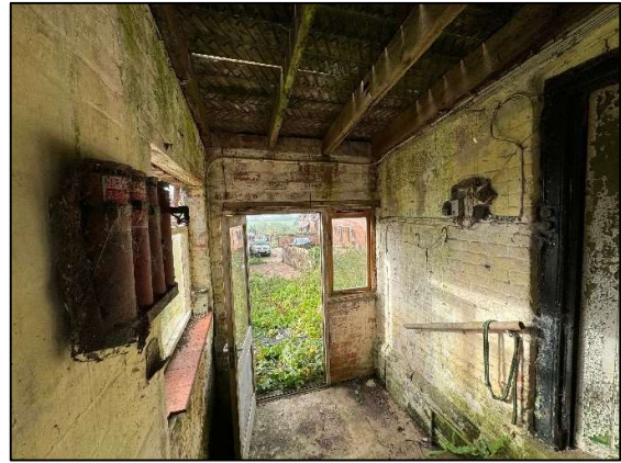
Photo 27: Internal View of Link Building
