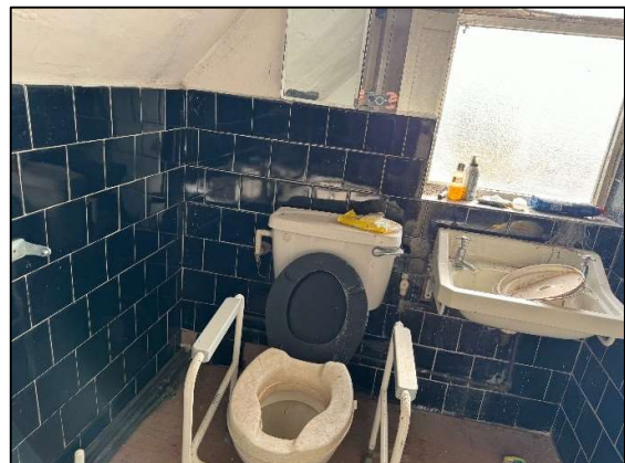
Photo 52: View of First Floor WC
