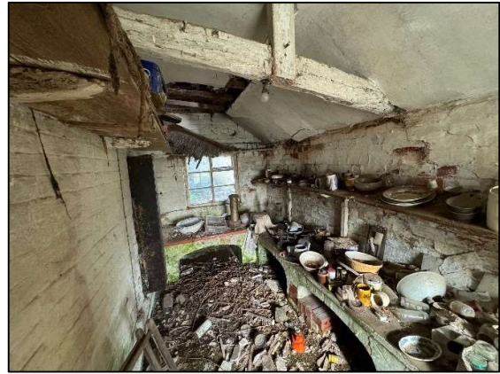
Photo 35: Internal View of Rear Extension
