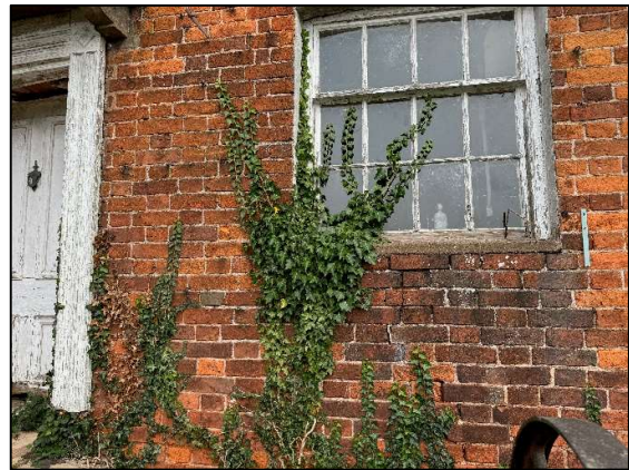
Photo 9: Vegetation Growth on Brickwork
