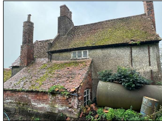
Photo 3: North Elevation of Farmhouse and Single Storey Rear Extension
