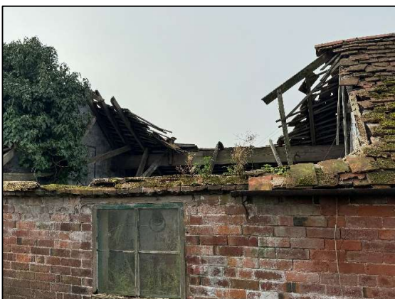
Photo 7: Part North Elevation of Adjoining Barn
