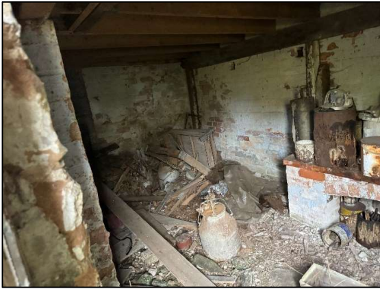
Photo 47: Internal View of Basement
