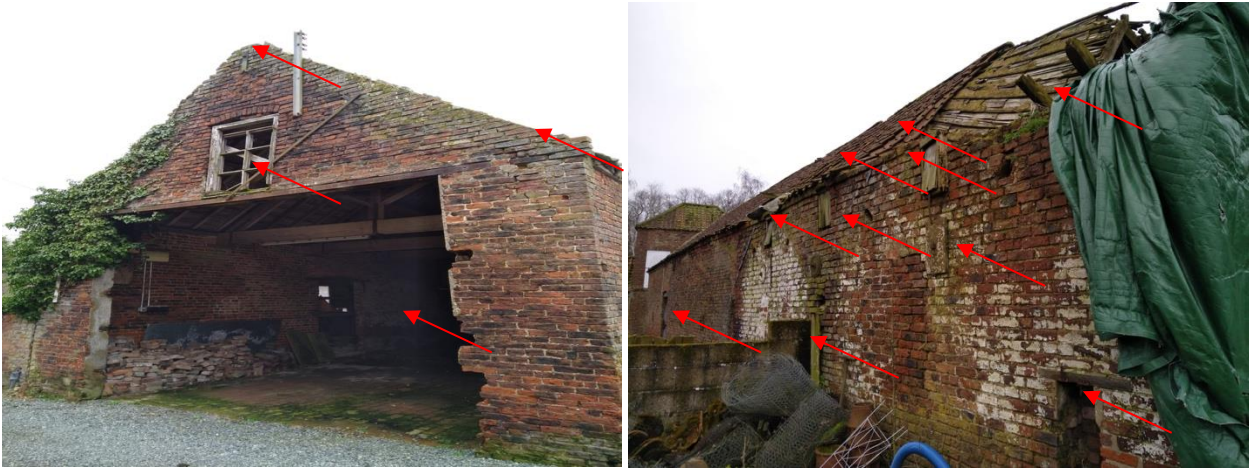
Plate 4.1 – (L) – Southern elevation, (R) – East elevation; highlighting potential access/roosting points
