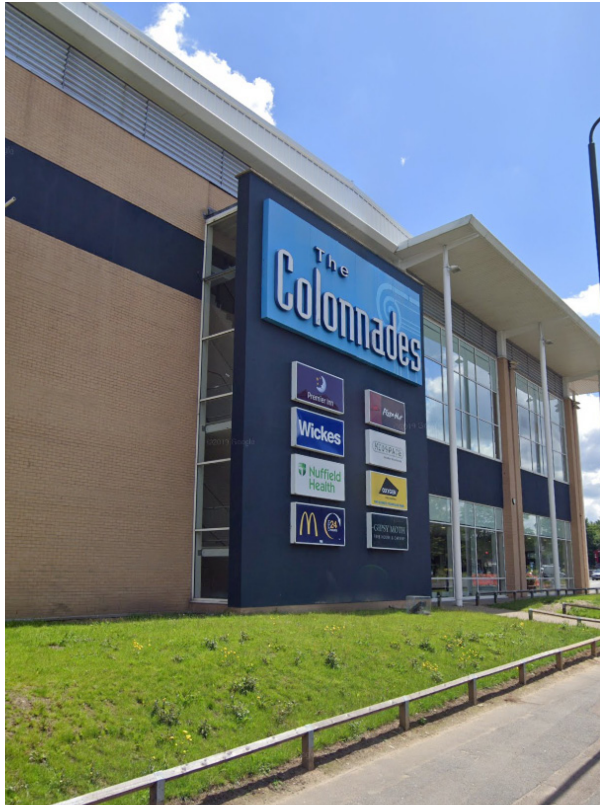
Existing wall signage viewed from Purley Way
