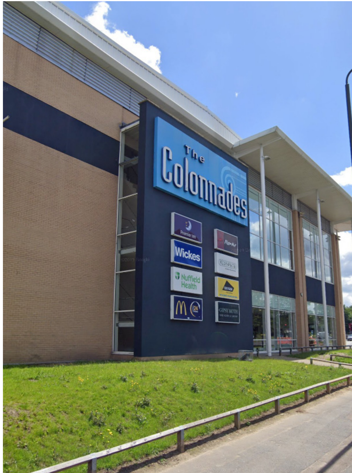
Existing wall signage viewed from Purley Way
