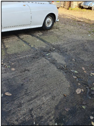
Figure 5 – tracks extended outside of shed to north west
