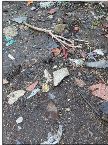
Figure 22 – suspected ACM at surface
