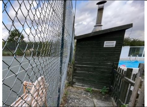
Photo 8. Pool house (shed)
