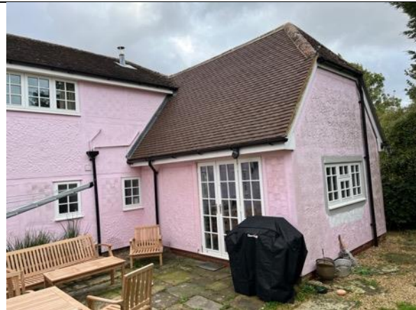
Photo 2. Rear of house (southwest section) showing area to be extended (wall with French doors and roof above). Note the relatively new roof tiles in immaculate condition
