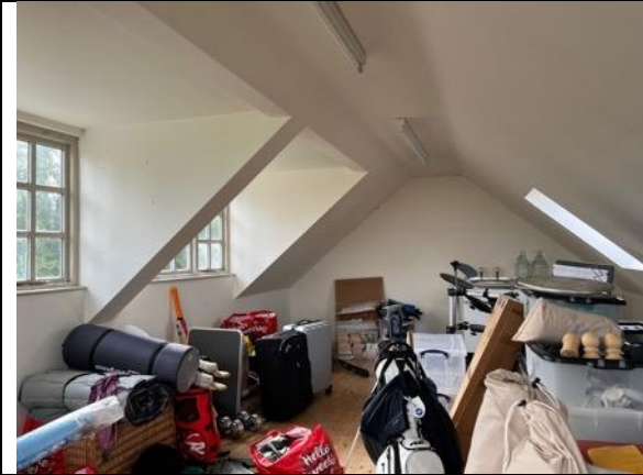
Photo 7. Interior of garage roof space
