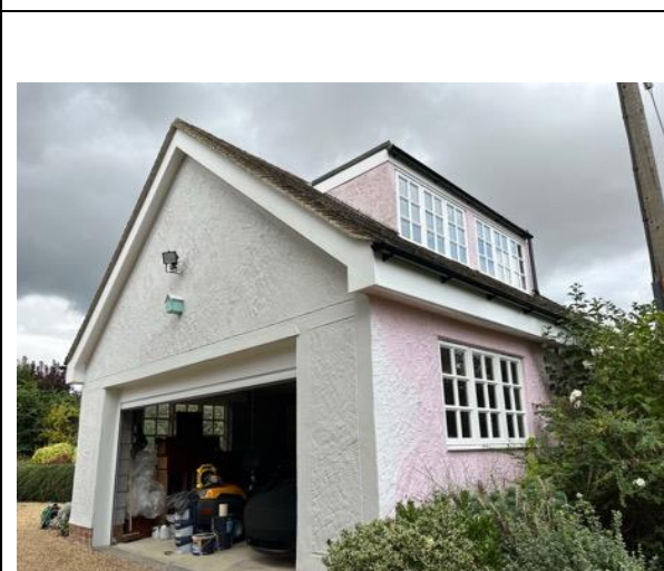
Photo 5. Detached garage to be converted to living space
