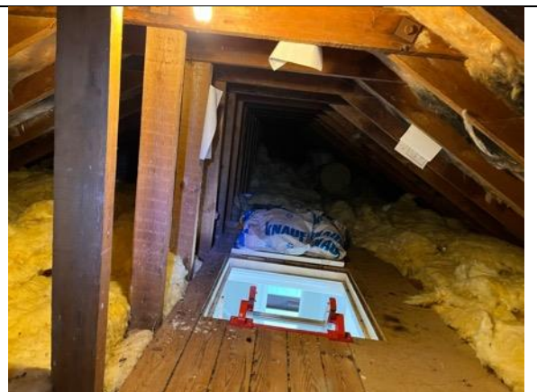
Photo 4. Roof space to house
