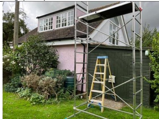
Photo 4. Garage from the northeast, showing north elevation with lean-to shed and tight-fitting soffit and fascia boards and roof tiles
