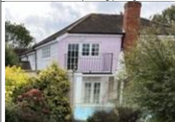
Photo 3. Balcony on north elevation to be replaced
