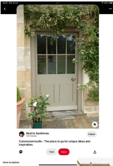
Example of timber door and frame
