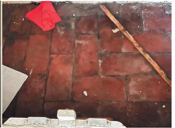
Original kitchen brick floor remaining visible within cupboard, intended to be revealed entirely for use in new utility room.
