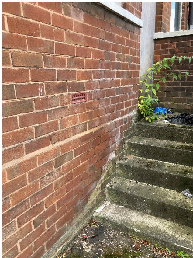
Figure 3.3: North East corner steps out of existing building.
