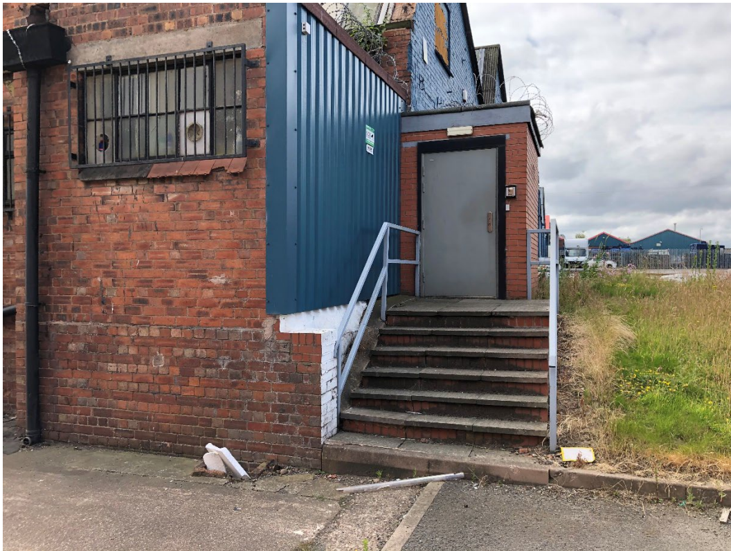
Figure 3.4: North West corner steps out of the existing building.
