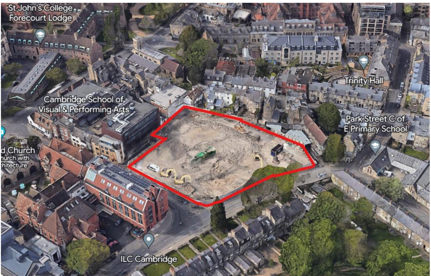
Figure 1: Site Location (Extracted from Google Earth)
