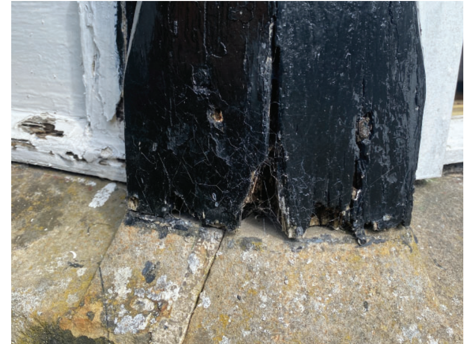
timber posts into stone cill
