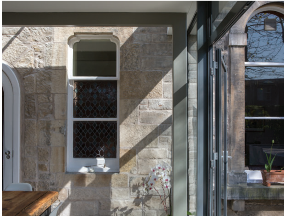
Example, existing external wall still legible in new extension, Trinity, Edinburgh
