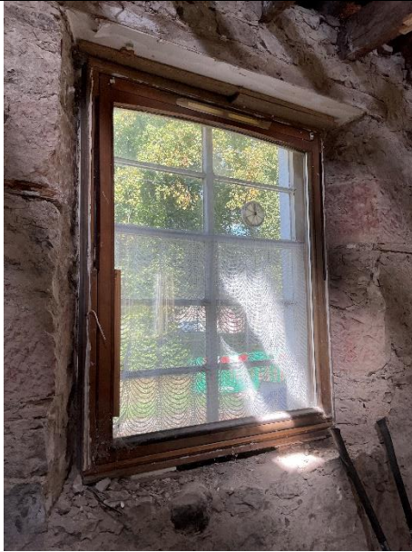
Internal view of GW01 (note: inner window is a reclaimed window installed backwards)
