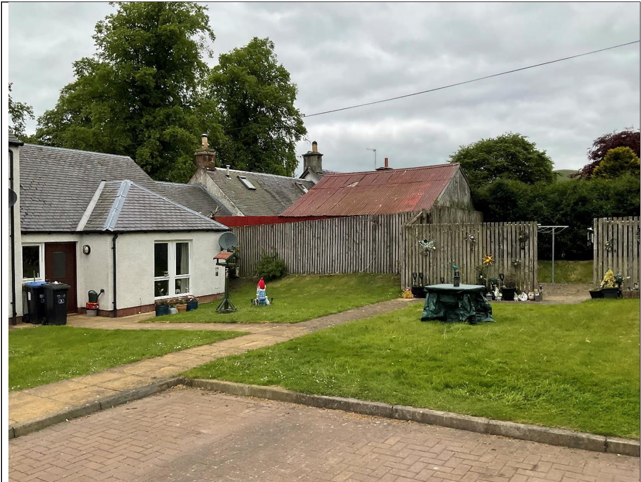
View of rear from The Limes showing existing fencing and shed
