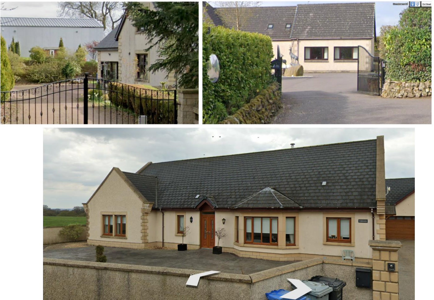
Figure 3: Existing house with vertical windows
