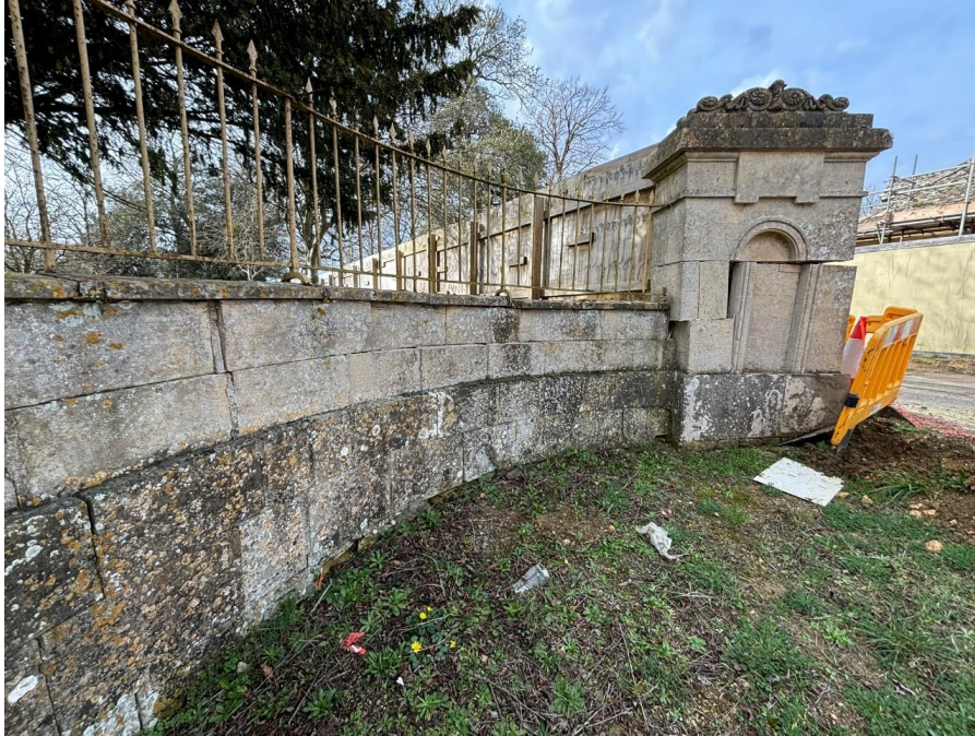
View from Road Side
