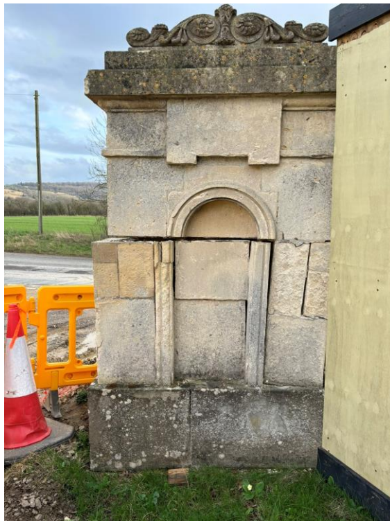
Pier from Estate Side
