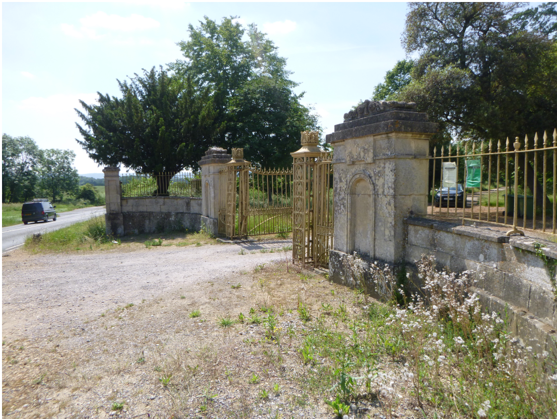
Figure 01 - Photo of existing gates, piers and adjoining walls from May 2021
