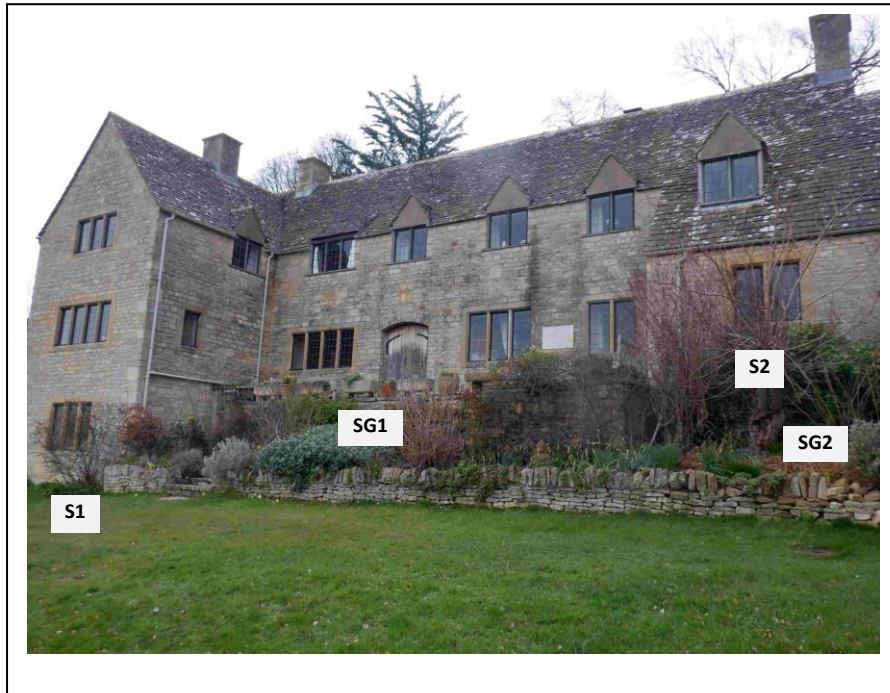
View of the rear elevation S1, S2, SG1 & SG2
