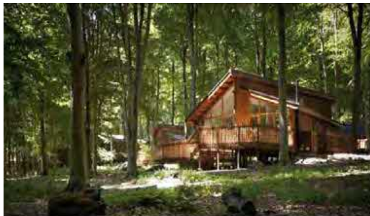
Fig 3. Typical finished chalet installation
