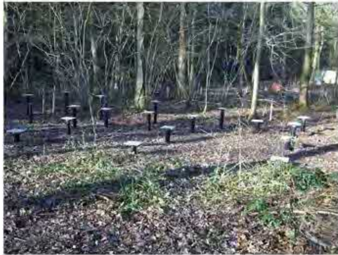
Fig 2. Example of Mini Piles in Forest of Dean - demonstrating minimal disruption to forest floor
