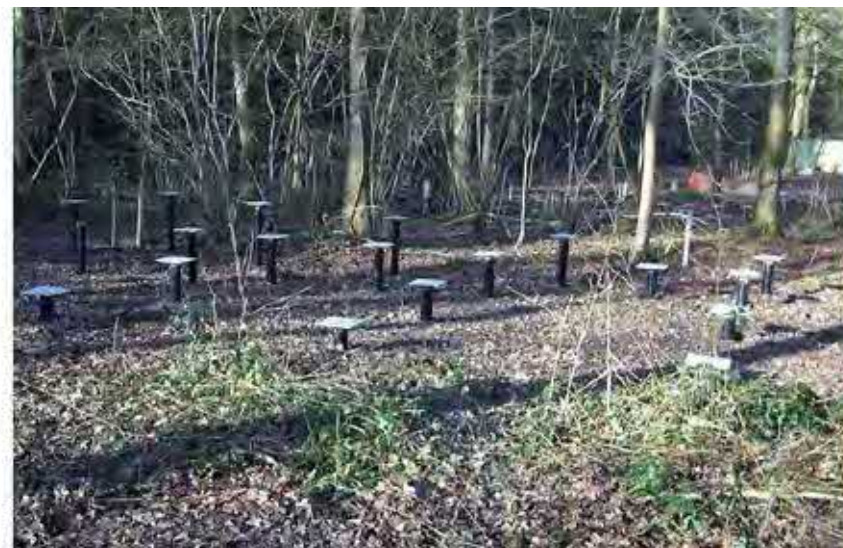
Fig 2. Example of Mini Piles in Forest of Dean – demonstrating minimal disruption to the forest floor.
