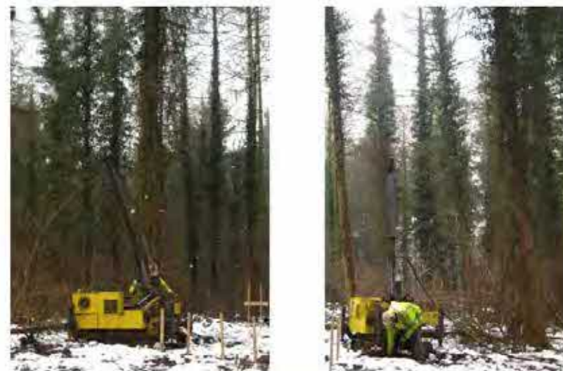
Fig1. Example of Mini Piling in the Forest of Dean
