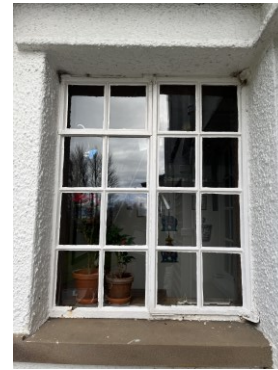
Steel crittall windows
