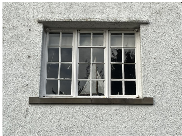
No. 19 - Existing Steel Crittall Style
