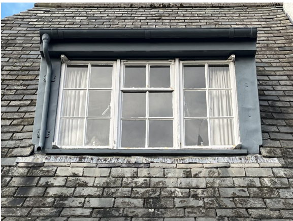
No. 18 - Existing Steel Crittall Style
