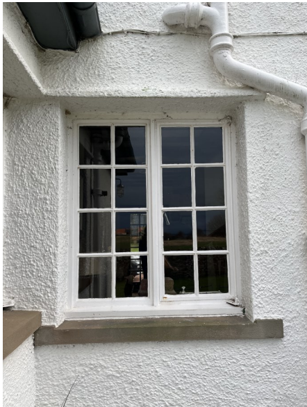
No. 12 - Existing Steel Crittall Style
