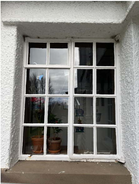
No. 11 - Existing Steel Crittall Style
