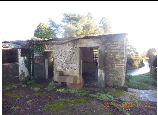
Plate 2. The western elevation of the stone stable
