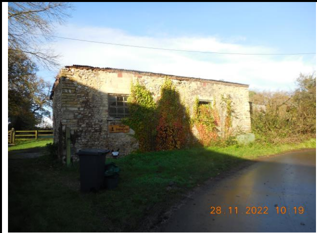
Plate 1. The eastern elevation of the stone stable
