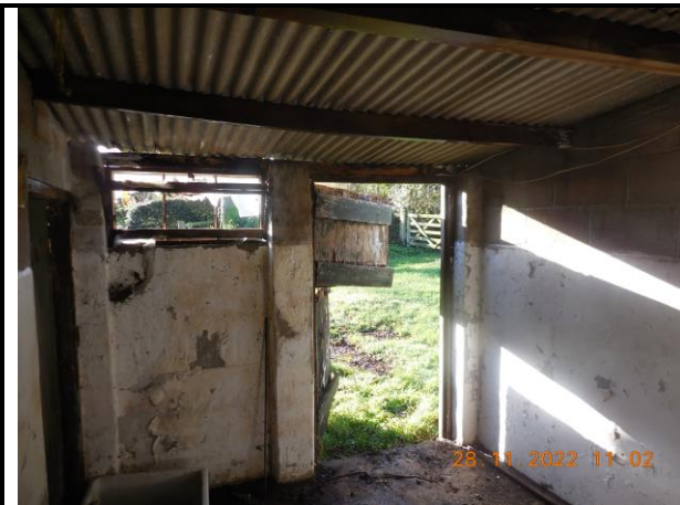
Plate 7. The interior of the storage shed
