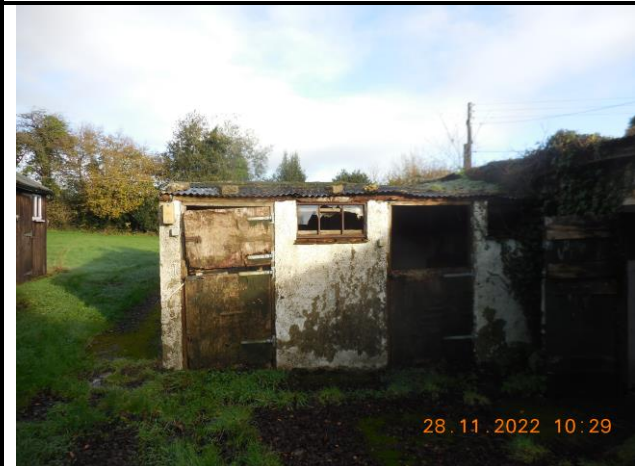
Plate 5. The southern elevation of the storage shed
