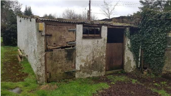
Figure 10. concrete block extension.
