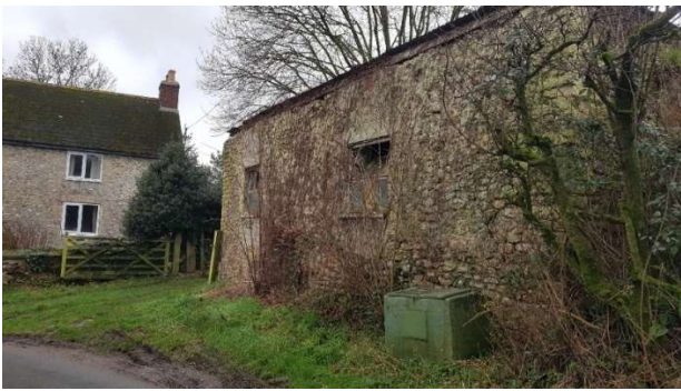
Figure 2. looking south from Alston. Farmhouse facing, stone building on right.
