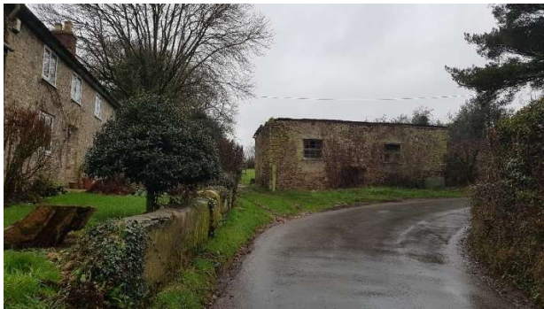
Figure 1. looking west from lane into Alston. Farmhouse on left, stone building facing.
