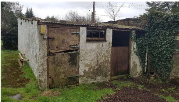
Figure 10. concrete block extension.
