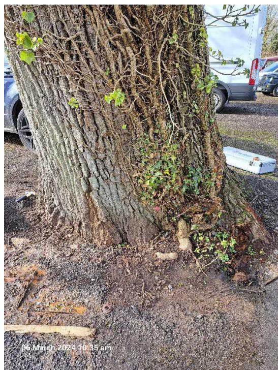
Drill point: East
