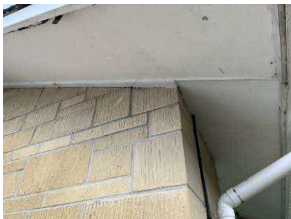
Photograph 6. Tightly fitted soffits.
