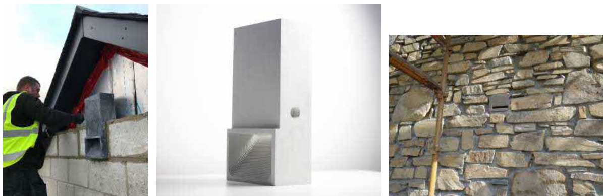
Photograph 10. 'Green and Blue' bat block and built in woodstone bat box `.
