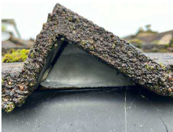
Photograph 7. Foam filler at eaves end of tiles.
