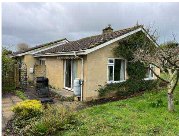
Photograph 2. East and north elevations.
