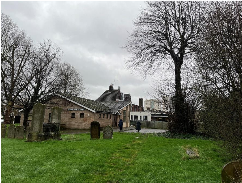
Figure 5: View of the building proposed for extension from the perspective of the churchyard.
