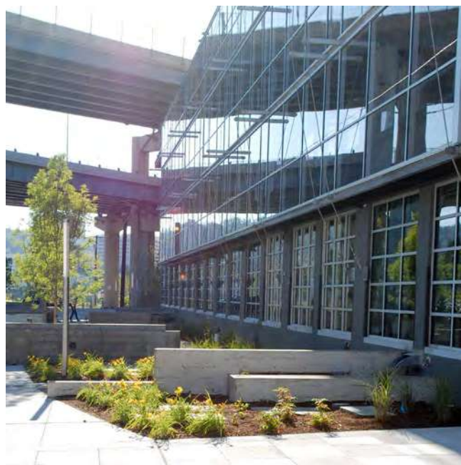
RiverEast Center, SE Portland
