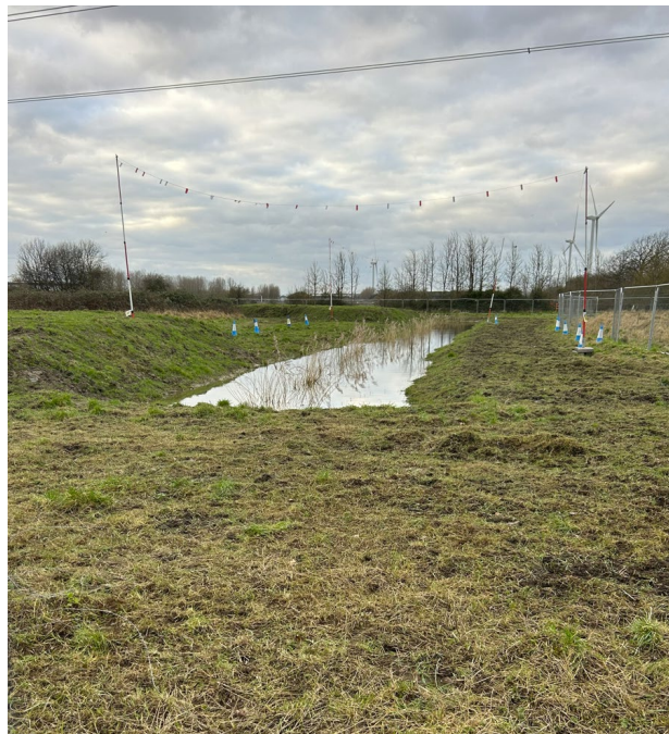
Figure 3: Ditch created in September 2023
