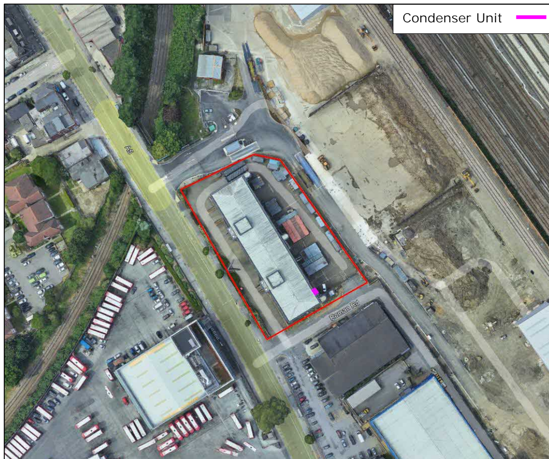
Figure 6-1: External condenser unit location
