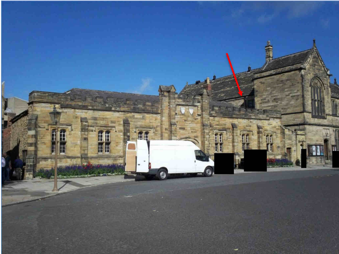
Photograph 1 – East and south elevations of The Education and Learning Centre. Red arrow shows roost location found in 2013
