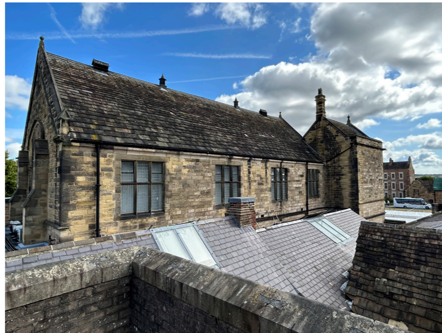
View of Wolfson Gallery from south
