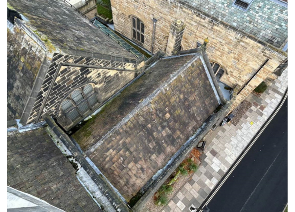
Palace Green Library roof (over Deane Room)
