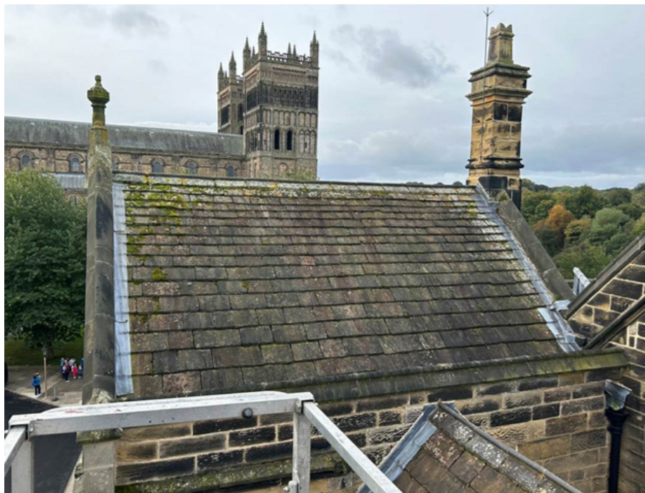
Palace Green Library roof (over stairwell looking south)
