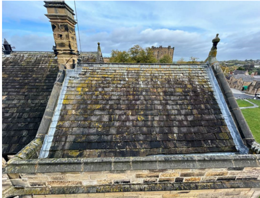
Palace Green Library roof (over stairwell looking north)
