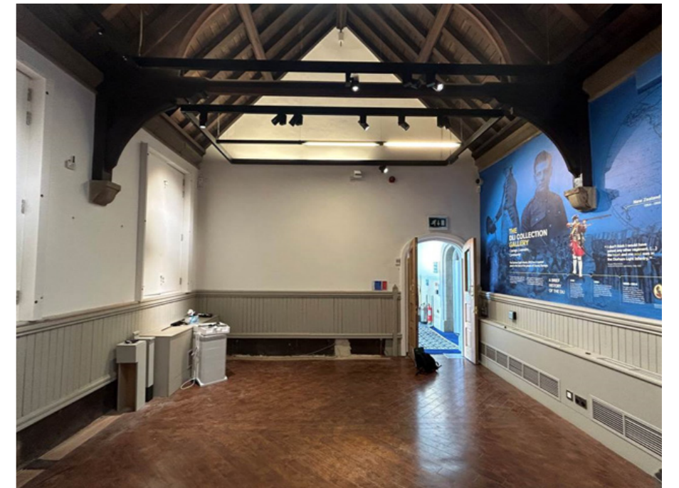
Underside of Deane Room roof
