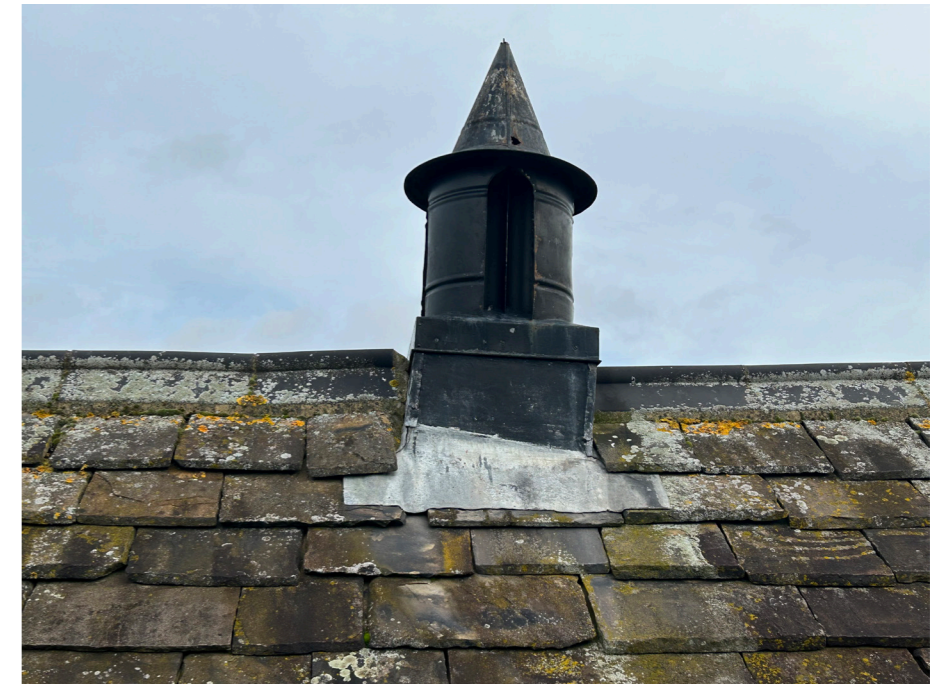
One of the 'witches hat' roof cowls
