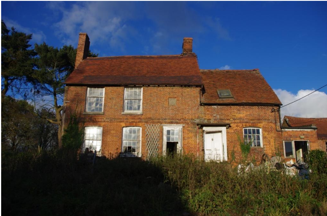
Figure 10 Building A Principal Elevation, General View (Looking North East).
