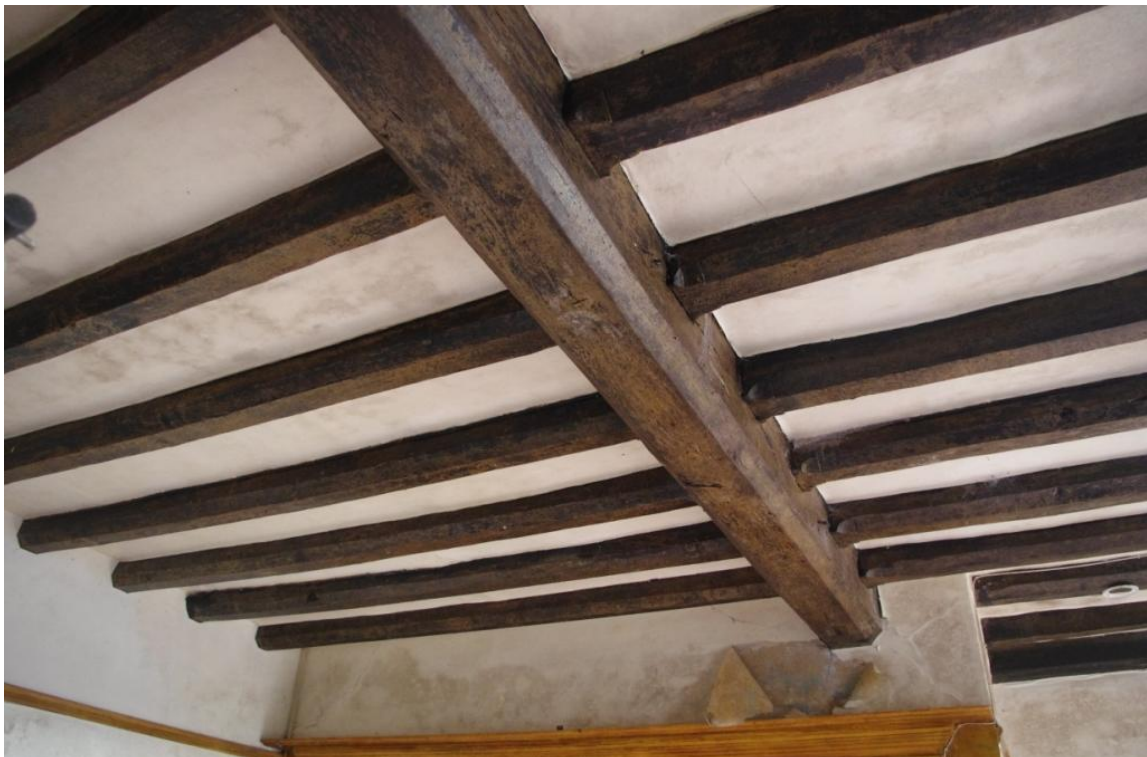
Figure 17 Building A (3) Ceiling Structure (Looking East – South East).
