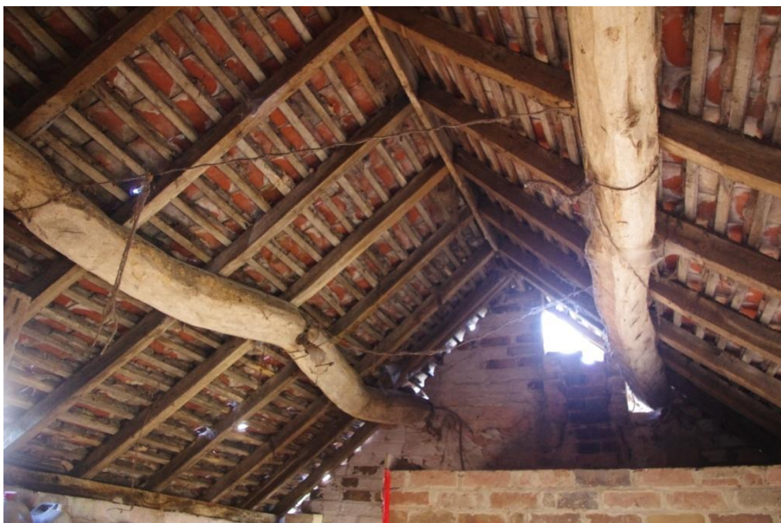
Figure 22 Building B (1) Roof Structure (Looking East).
