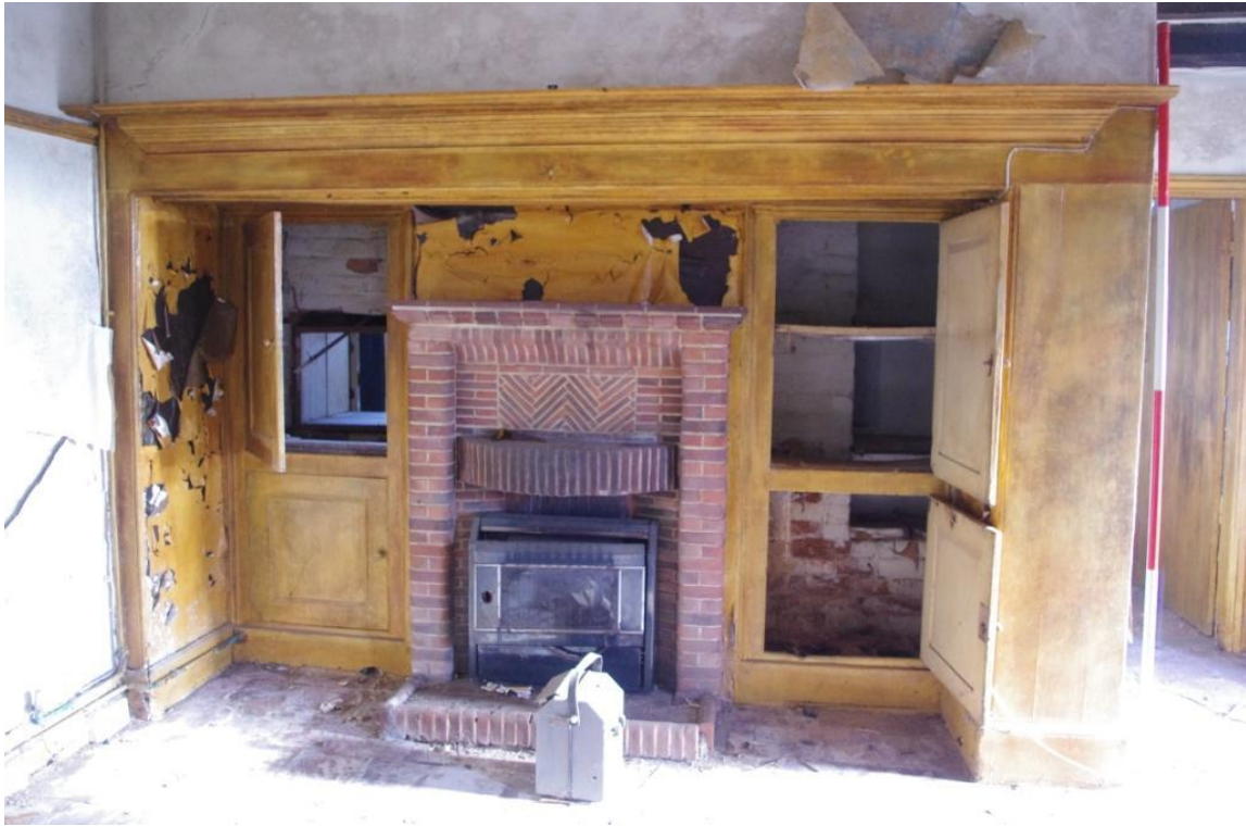
Figure 16 Building A (3) Inglenook Fireplace (Looking East – South East).
