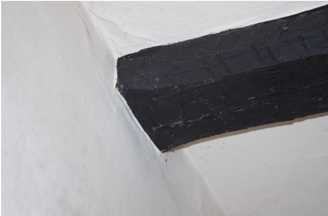
Figure 19 Building A (11) Runout Stopped Collar Purlin (Looking North).
