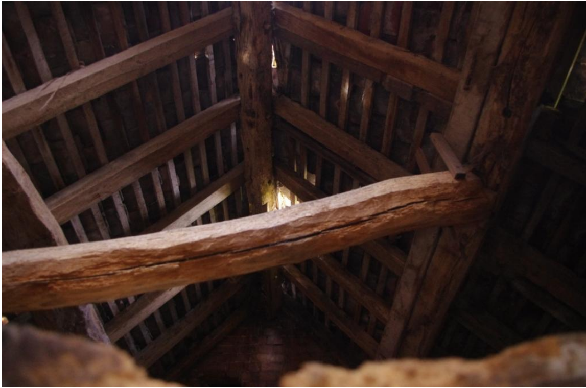
Figure 20 Building A Limited View of Roof Structure (Looking North West).
