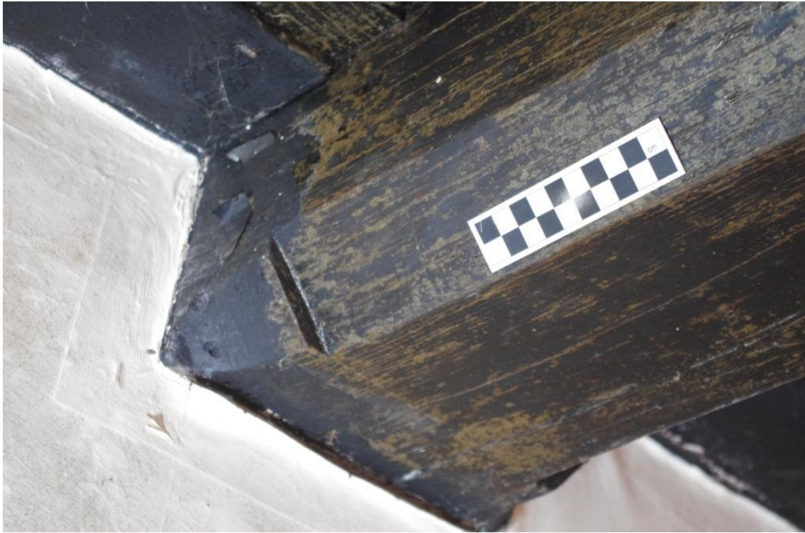
Figure 18 Building A (3) Step & Runout (Looking North).
