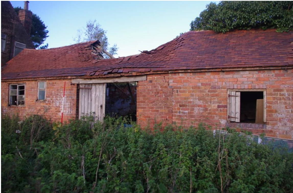
Figure 21 Building B Principal Elevation (Looking West – North West).
