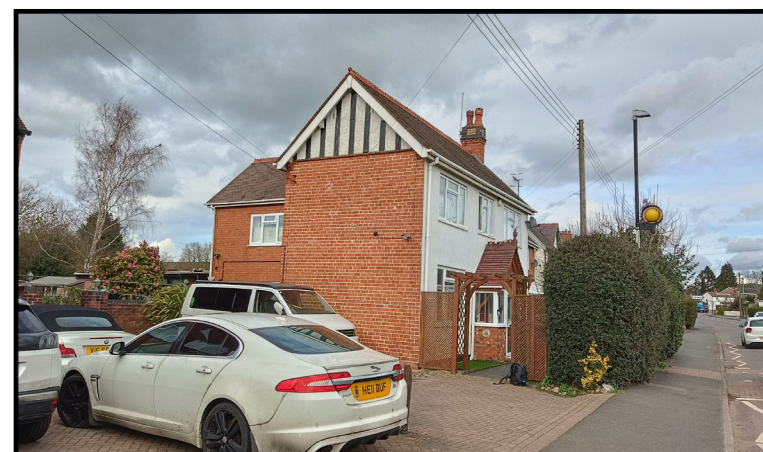
REAR ELEVATION PHOTOGRAPH
