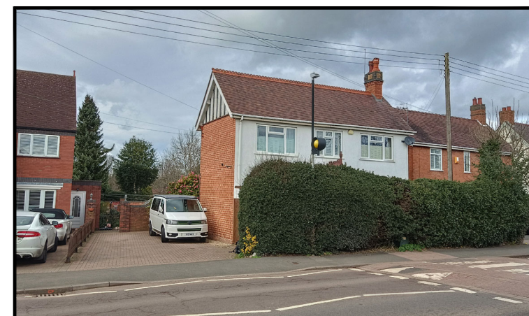
FRONT ELEVATION PHOTOGRAPH
