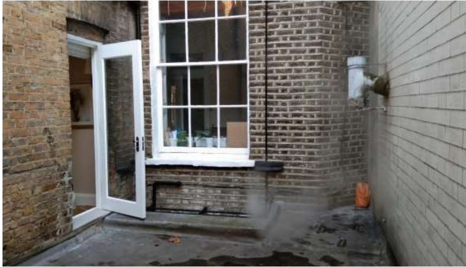
ABOVE: new doorway exiting the living room in order to access the flat roof over the bedrooms of Flat 2, the window serves the kitchen.
