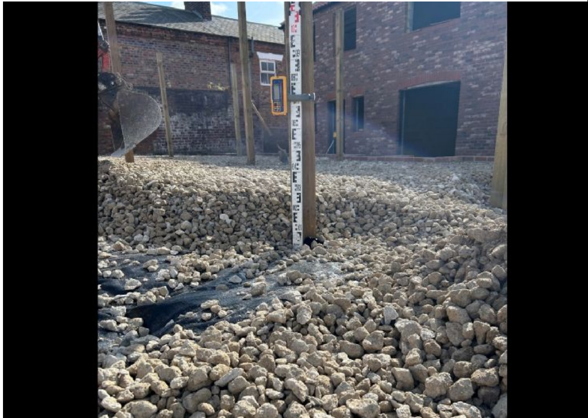
Hardstanding placement – plots 1 to 4
