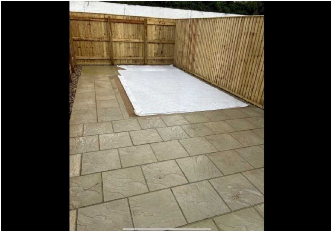
Artificial grass membrane (before placement of artificial grass)
