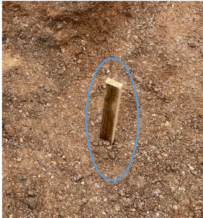
Initial site strip reference point
