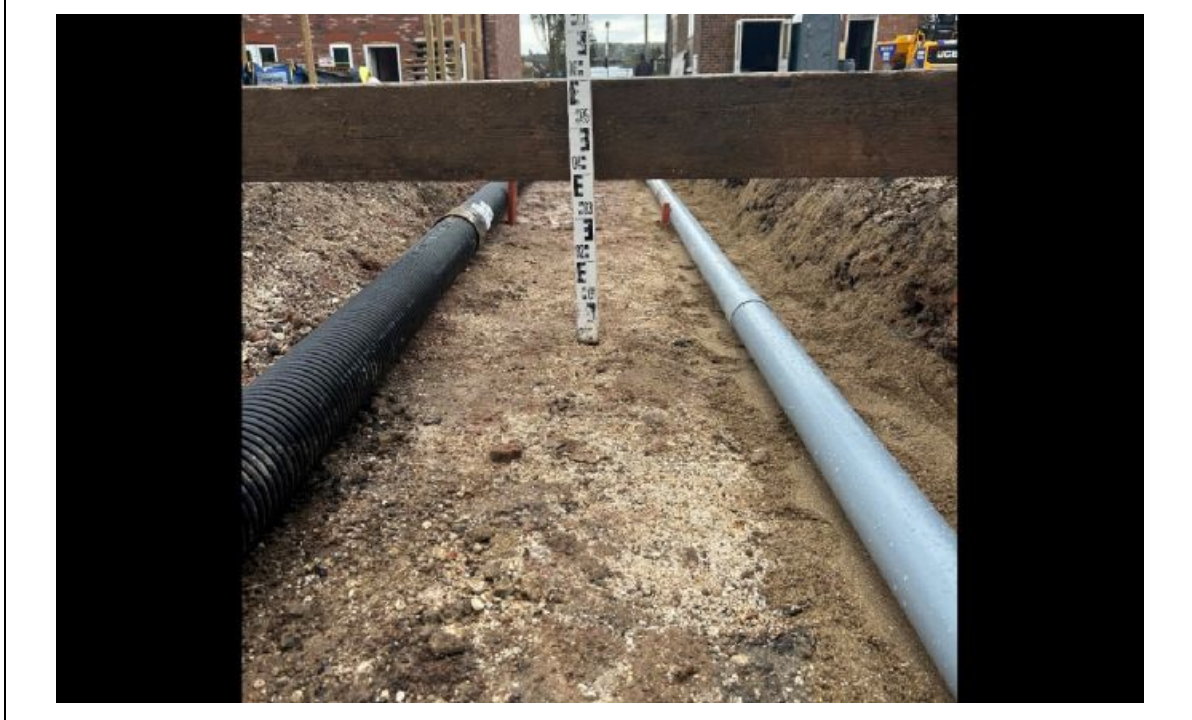
Evidence of trenches to pipe installation
