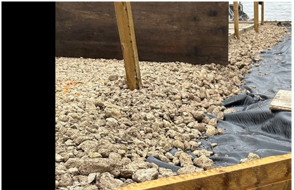
Hardstanding placement – plots 7 and 8
