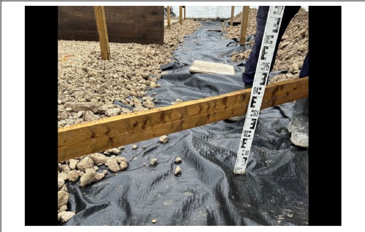
Evidence of membrane – plots 1 to 4
