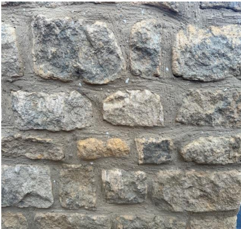
External Wall Site Sample Panel: Lime Mortar Pointing
