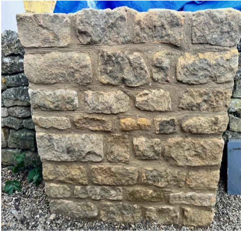
External Wall Site Sample Panel
