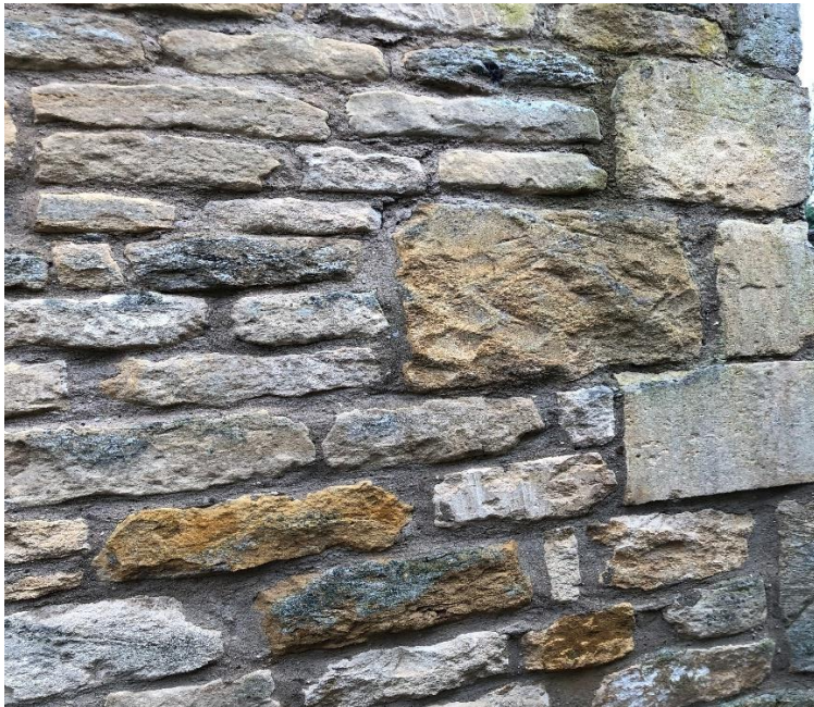
External Wall: Natural Stone in Lime Mortar
