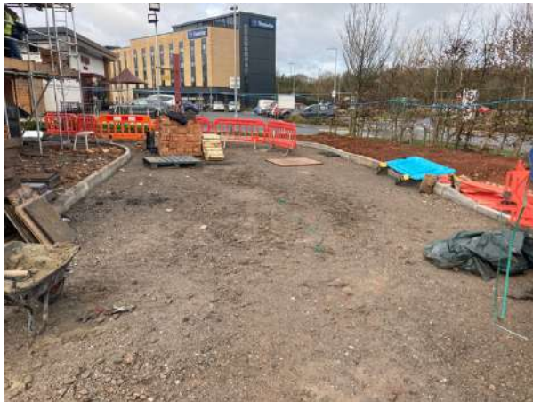
Photo 9: Construction of roadway around Greggs unit on 16 th February 2024
