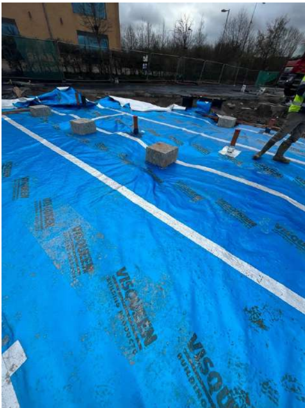
Photos 9 & 10 – PCA supplied photos showing all joints and service entries have been sealed.
