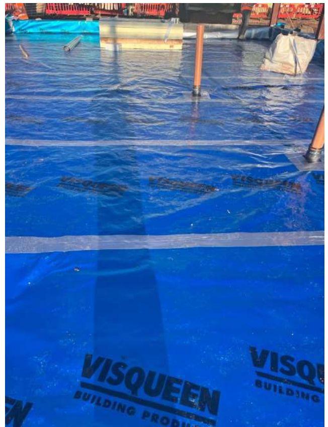
Photos 9 and 10 – PCA supplied photo showing all joints to have been sealed.
