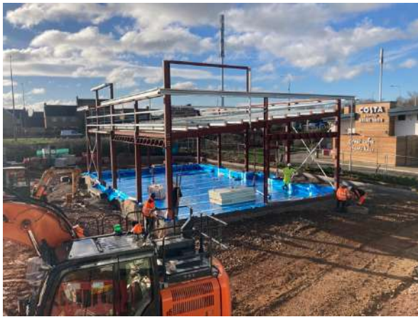
Photo 5: View south-westwards towards Greggs retail unit on 10 th January 2024.
