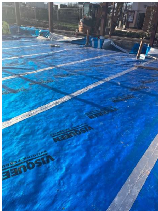
Photos 11 and 12 – PCA supplied photo showing all joints to have been sealed, and top hat covers installed.
