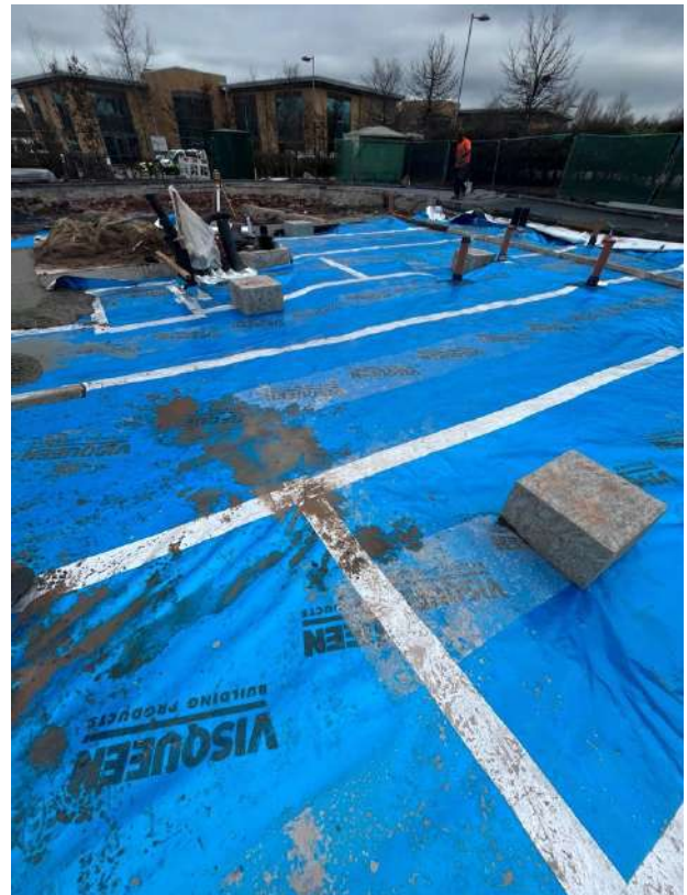
Photos 9 & 10 – PCA supplied photos showing all joints and service entries have been sealed.
