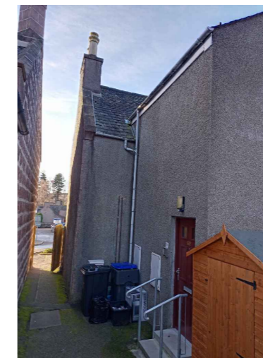
Existing Door At Side Elevation
