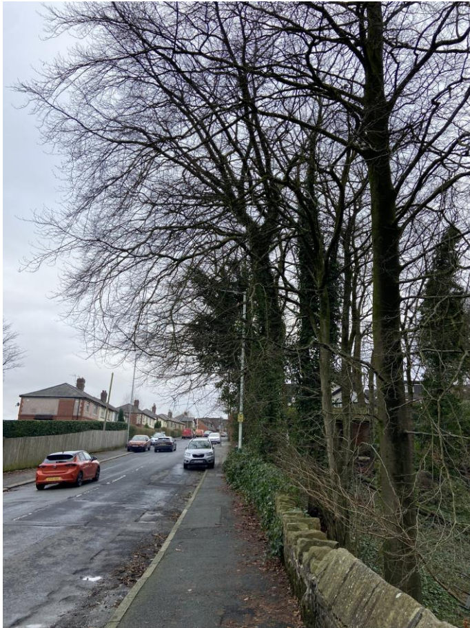
Image 9 – indicating T6 – T13 overhanging highway and pathway – request for crown lift to create sufficient vehicular and pedestrian clearance
