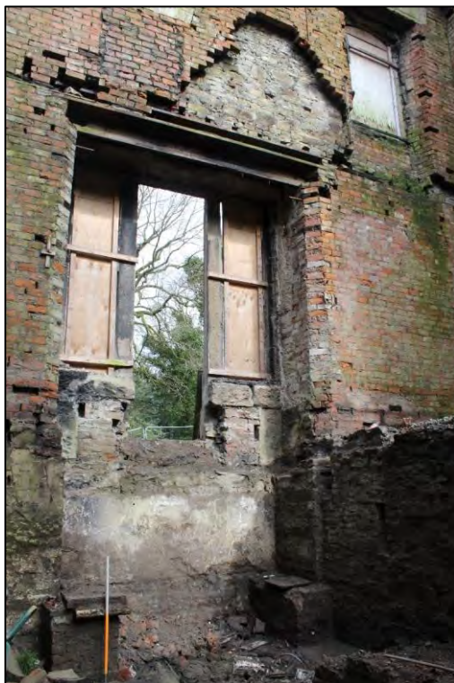
Plate 25: Internal view looking NE within the basement
