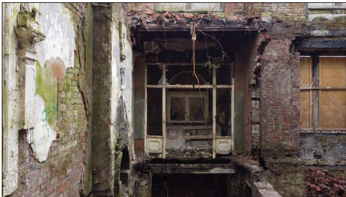
Plate 34: Internal view looking W towards the main entrance with the entrance hall at ground floor level
