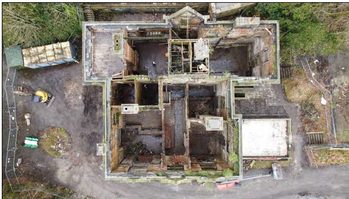
Plate 2: Aerial view of Horncliffe Mansion showing the extent of the internal fire damage
