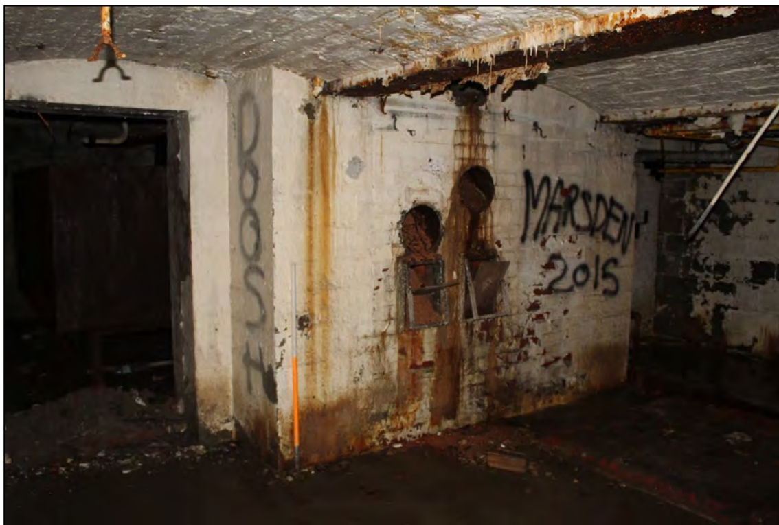
Plate 30: Internal view looking NE within the basement
