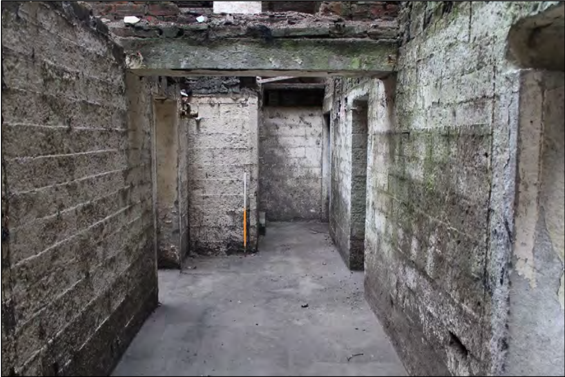
Plate 26: Internal view looking N within the basement corridor
