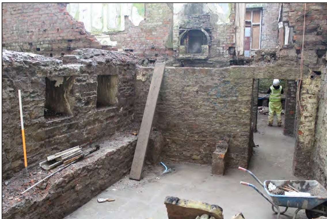
Plate 23: Internal view looking SSE within the basement
