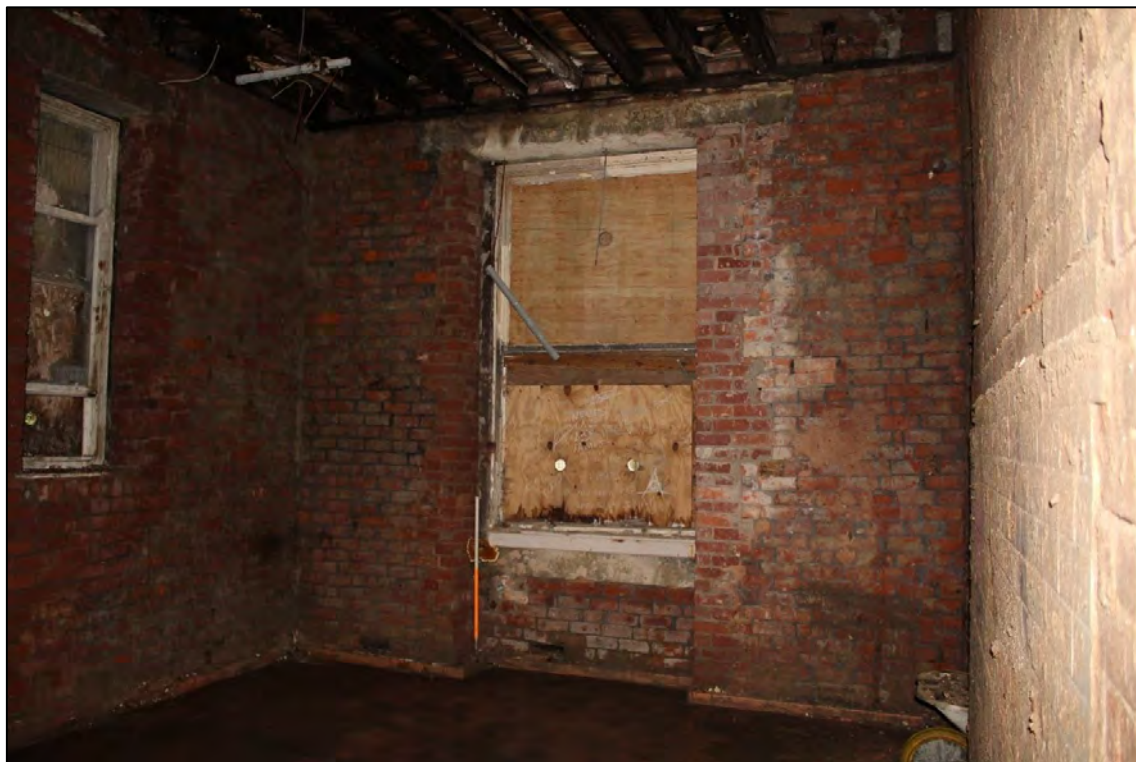
Plate 47: Internal view looking E within a ground floor service compartment
