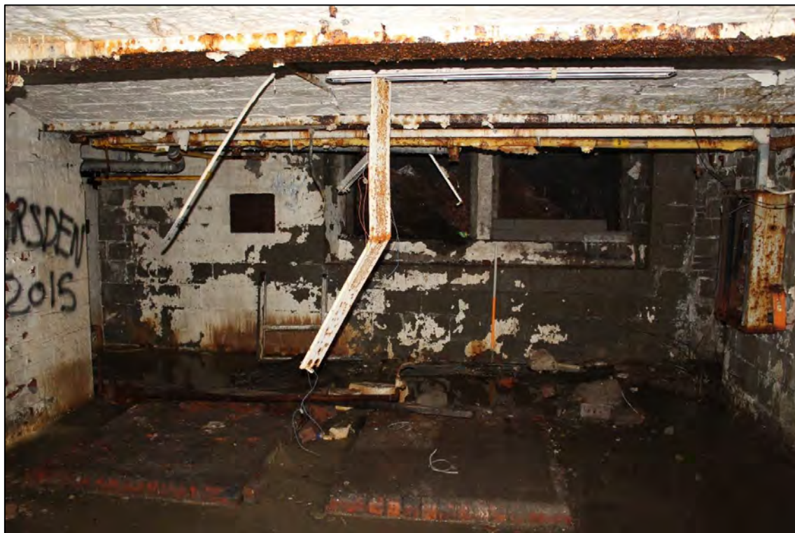
Plate 29: Internal view looking E within the basement
