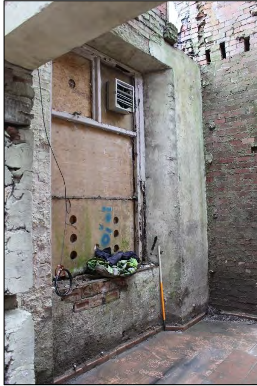
Plate 57: Internal view looking SE within a ground floor service compartment
