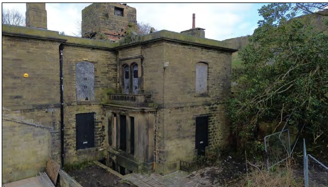
Plate 10: View looking NE towards the southern elevation
