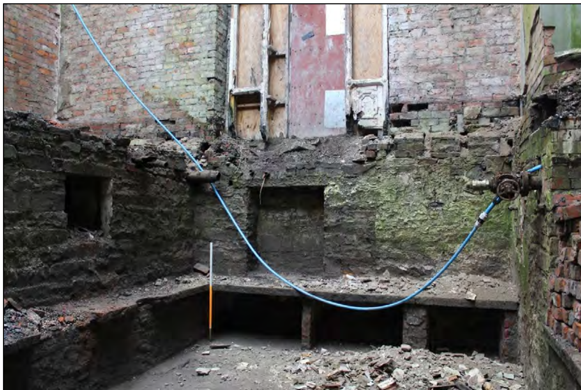
Plate 21: Internal view looking S within the basement
