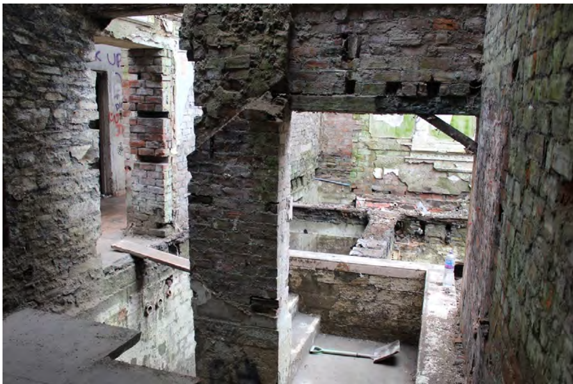
Plate 52: Internal view looking SE within a ground floor service compartment
