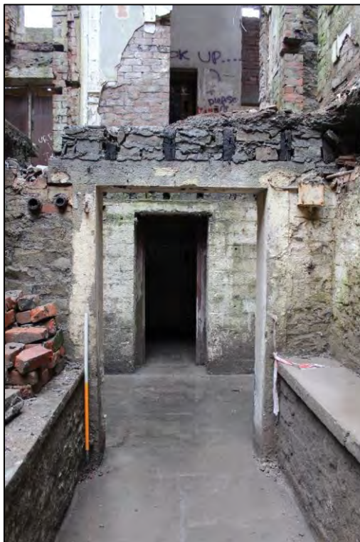
Plate 20: Internal view looking E towards the doorway within the eastern end of the central corridor with the basement
