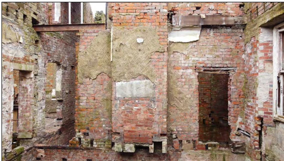
Plate 92: View looking N at first floor level
