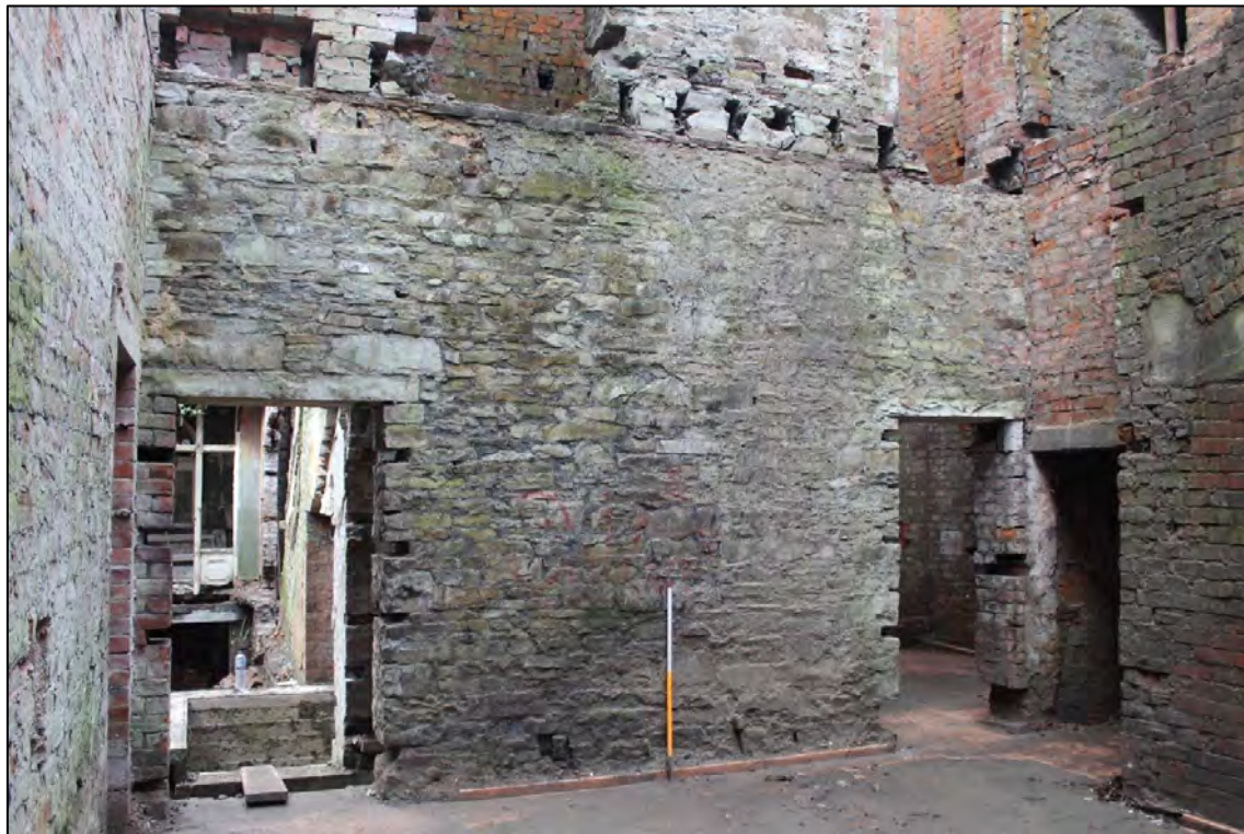
Plate 55: Internal view looking W within a ground floor service compartment
