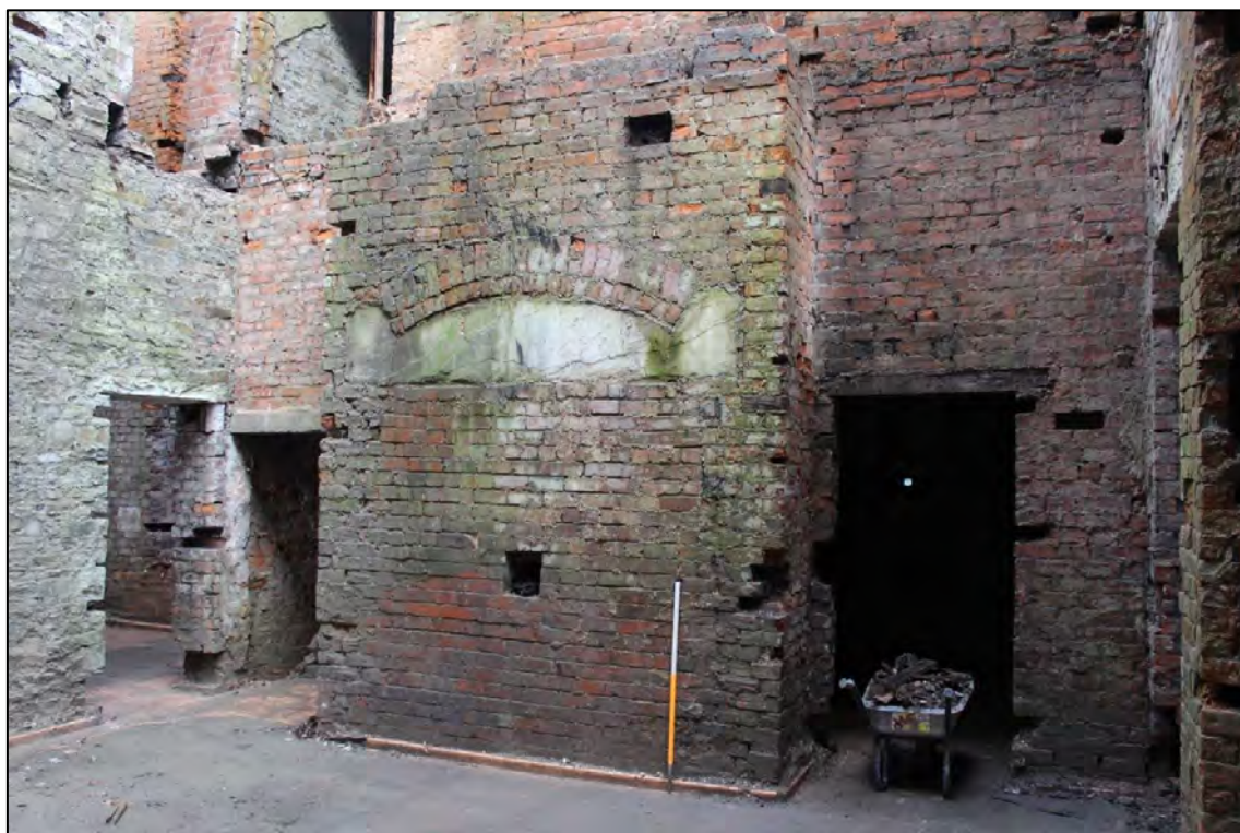
Plate 54: Internal view looking N within a ground floor service compartment
