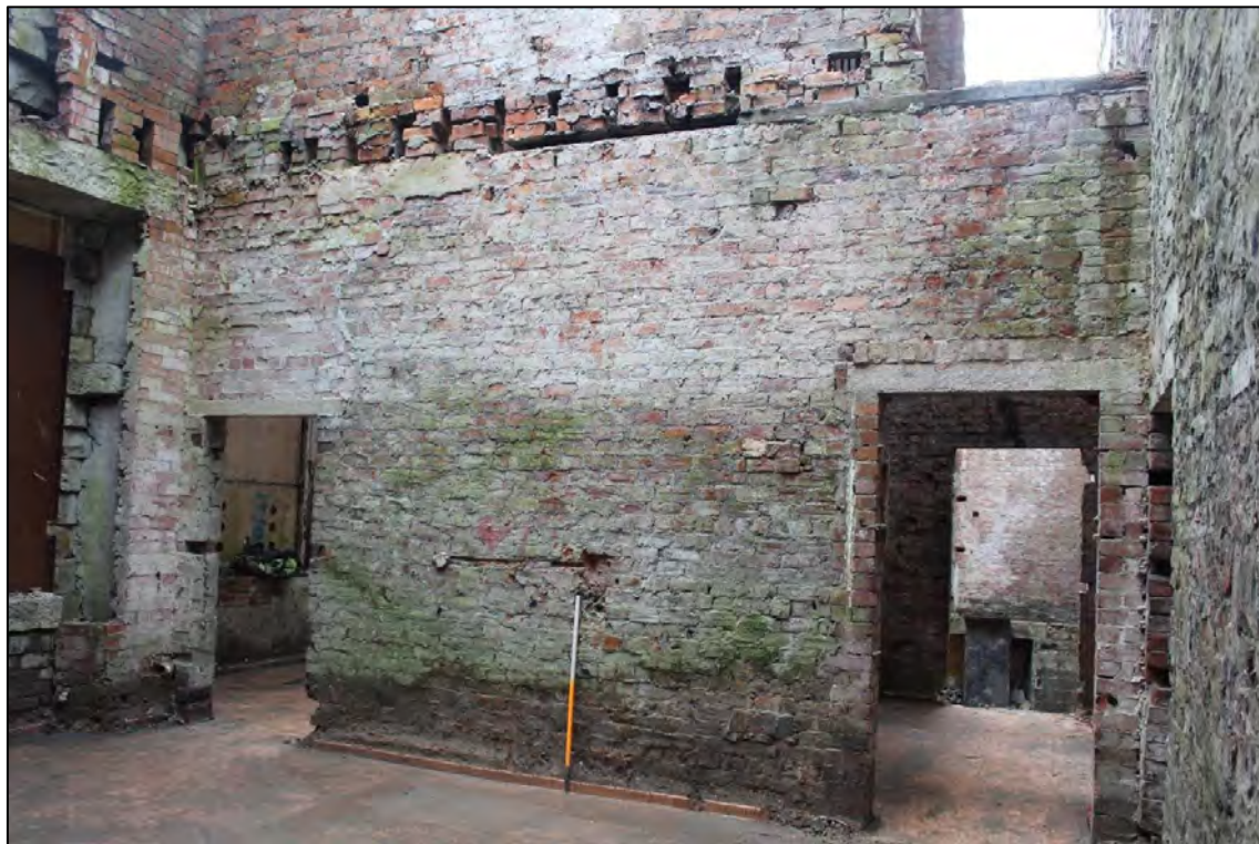
Plate 56: Internal view looking S within a ground floor service compartment
