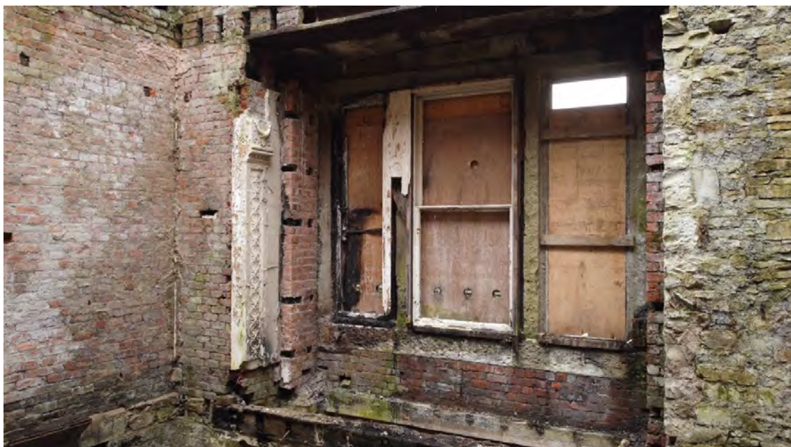
Plate 60: Internal view looking WSW within a ground floor living compartment
