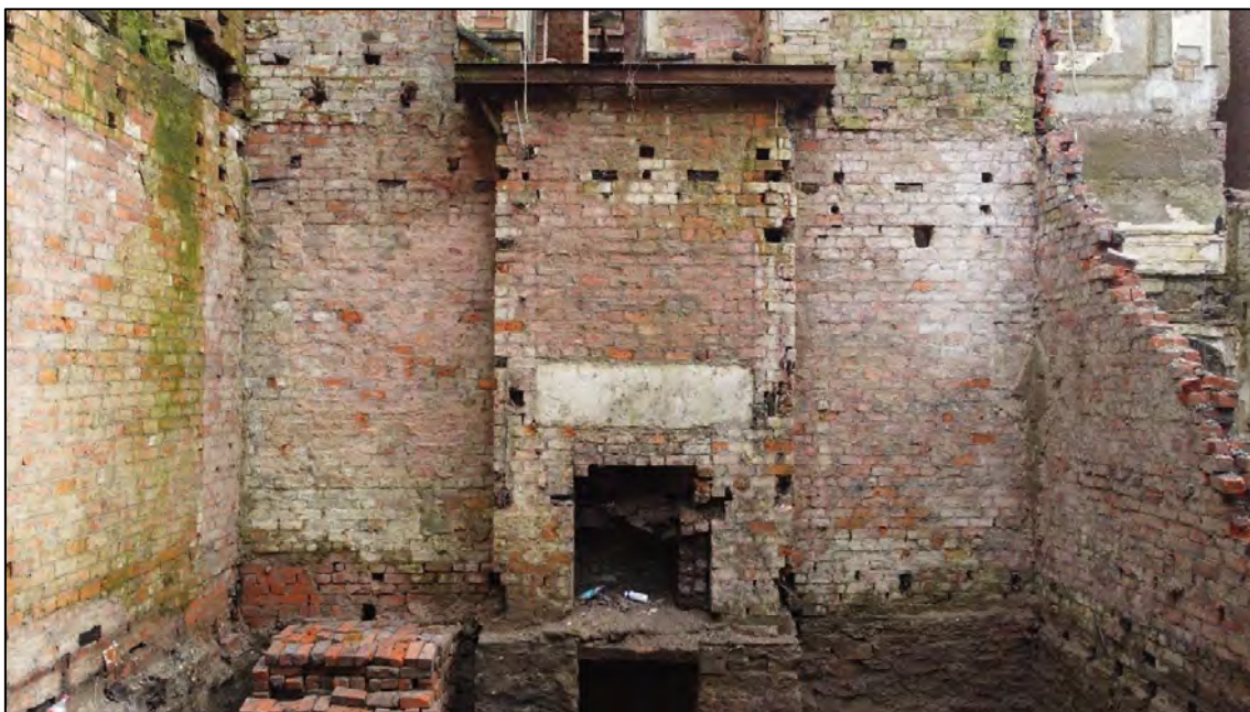
Plate 36: Internal view looking E within one of the principal living compartments at ground floor level
