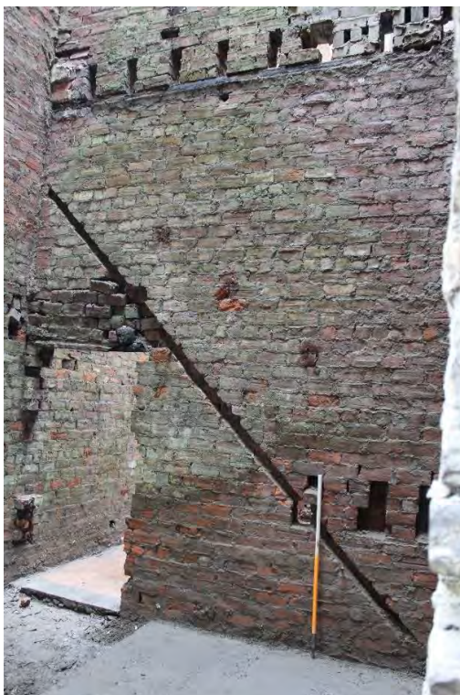
Plate 51: Internal view looking NW within a ground floor service compartment
