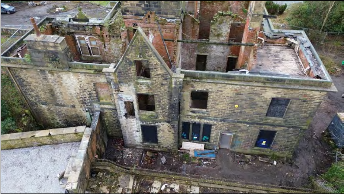
Plate 13: View looking W towards the rear E facing elevation
