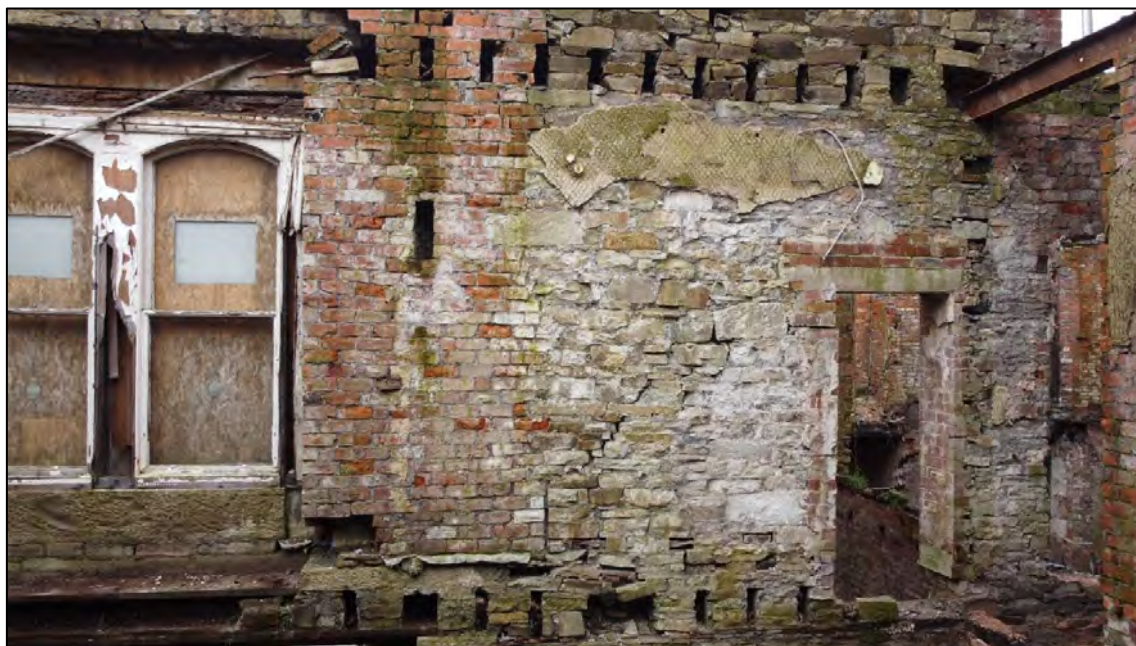
Plate 91: View looking W at first floor level
