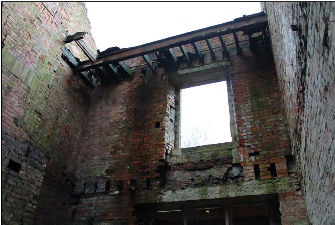
Plate 81: View looking E at first floor level
