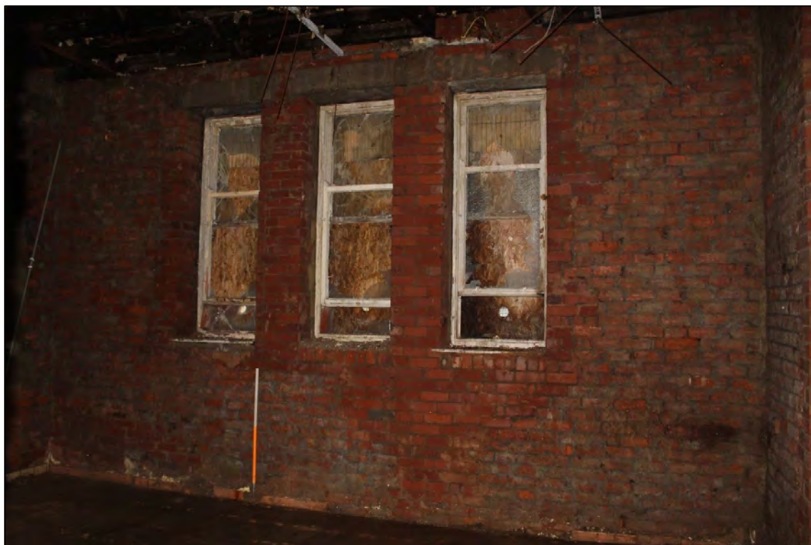
Plate 48: Internal view looking N within a ground floor service compartment
