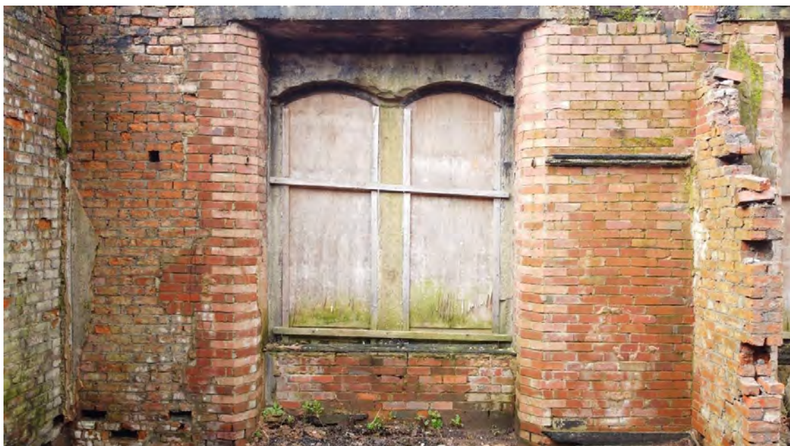
Plate 74: Internal view looking W at first floor level
