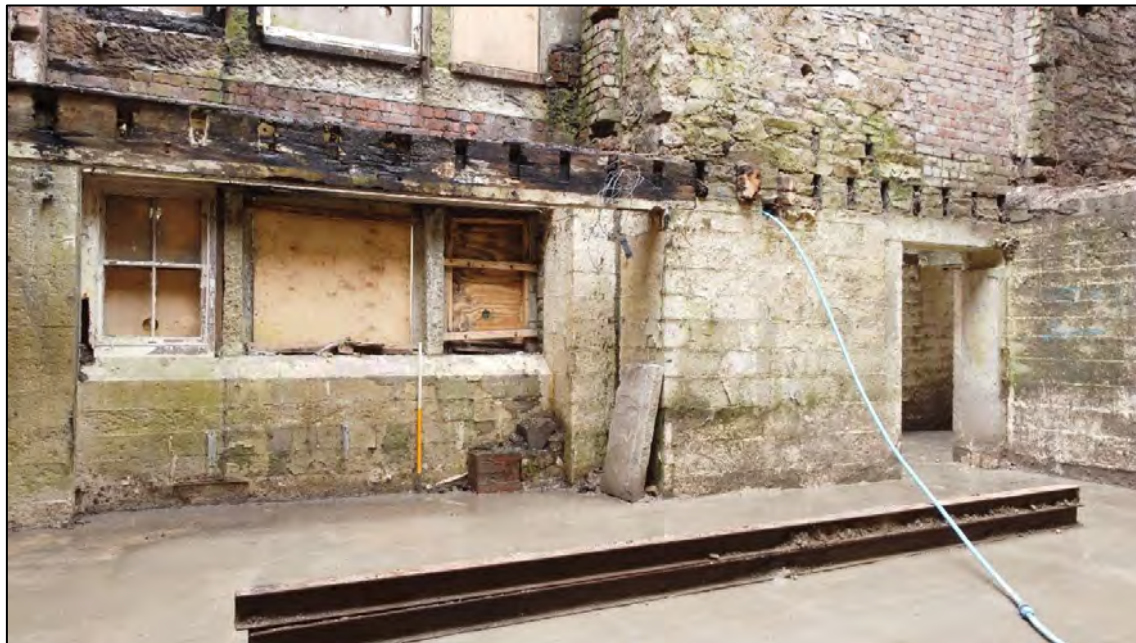
Plate 33: Internal view looking WNW within the basement
