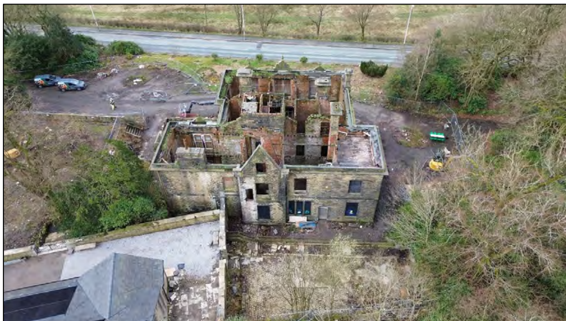
Plate 7: View looking W towards the rear elevation
