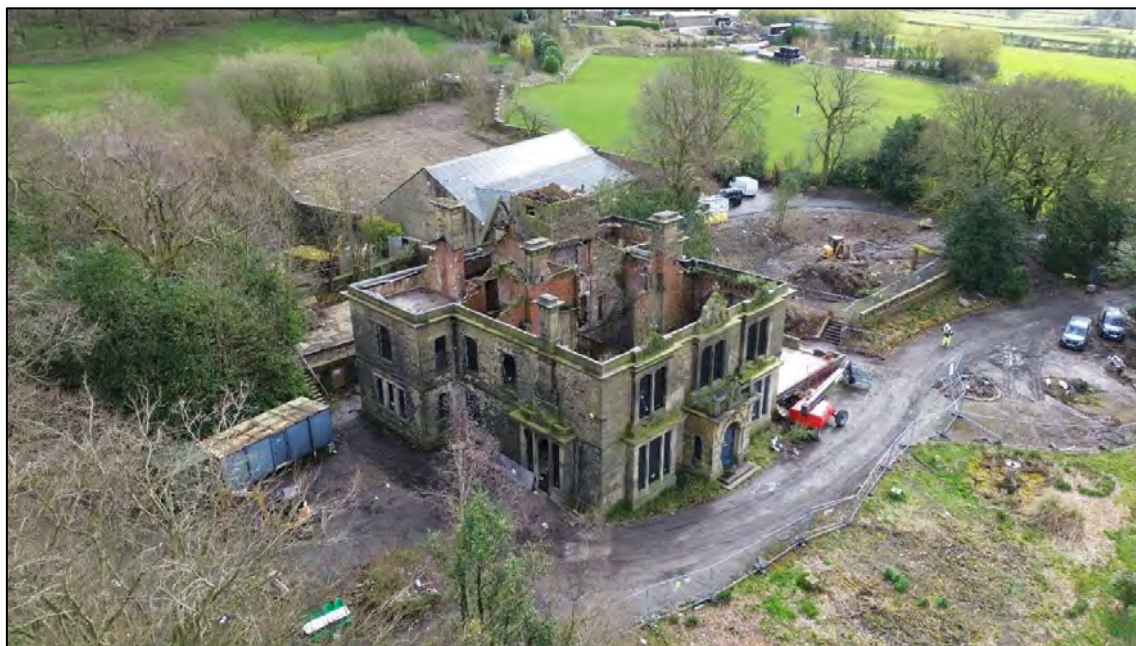
Plate 6: View looking SE towards the principal W facing elevation
