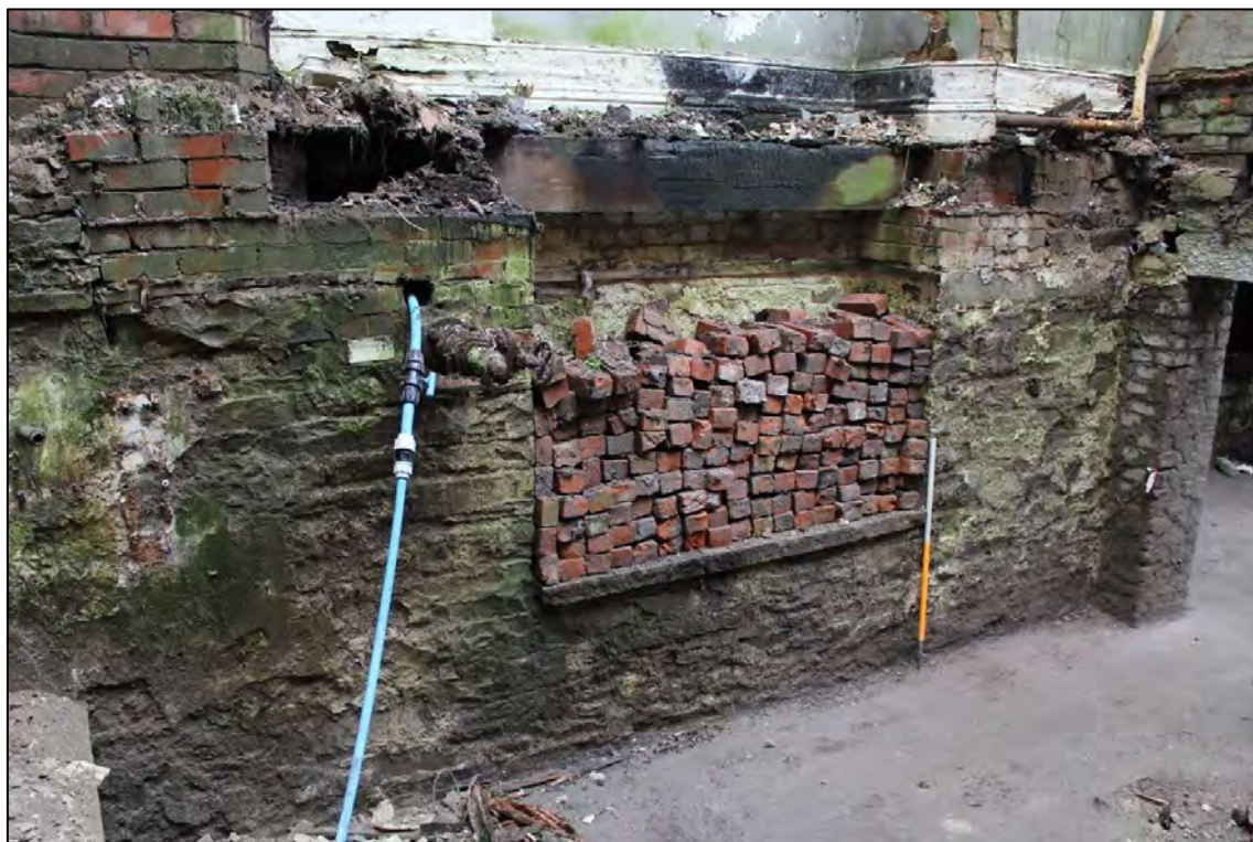
Plate 22: Internal view looking NW within the basement
