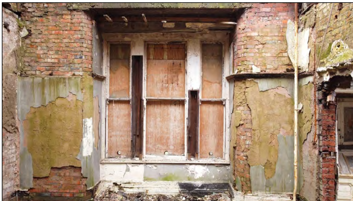
Plate 42: Internal view looking W within one of the principal living compartments at ground floor level
