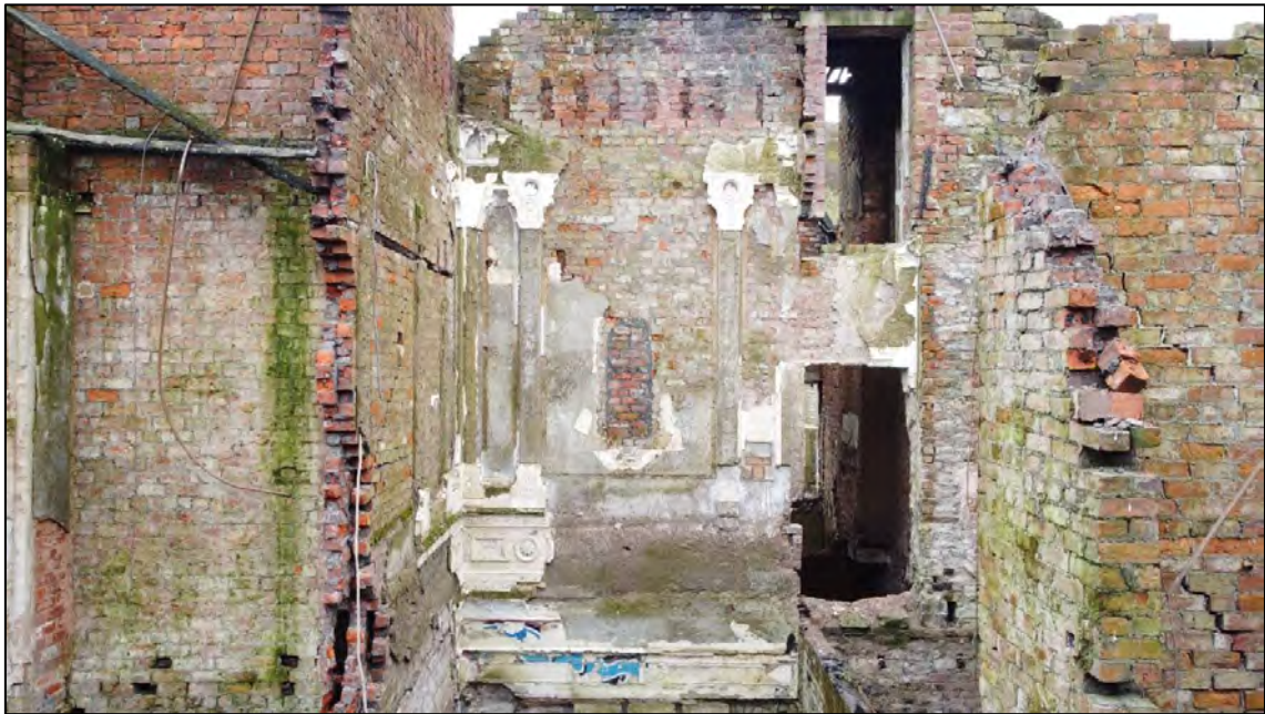
Plate 76: Internal view looking E at first floor level in the location of the former stairs landing
