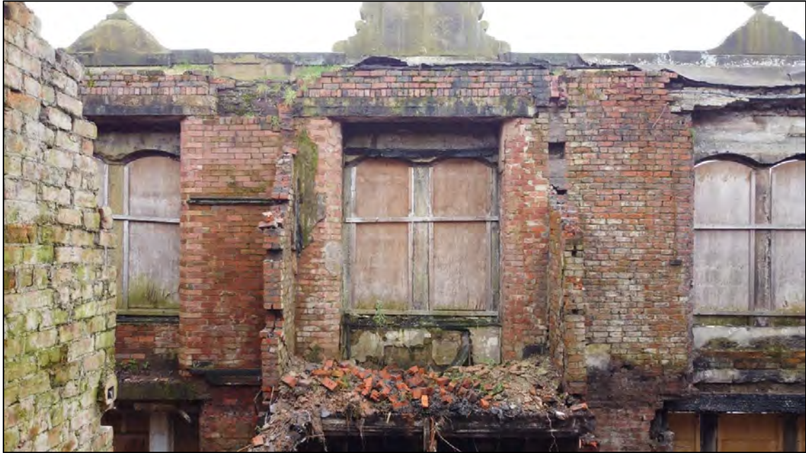
Plate 75: Internal view looking W at first floor level
