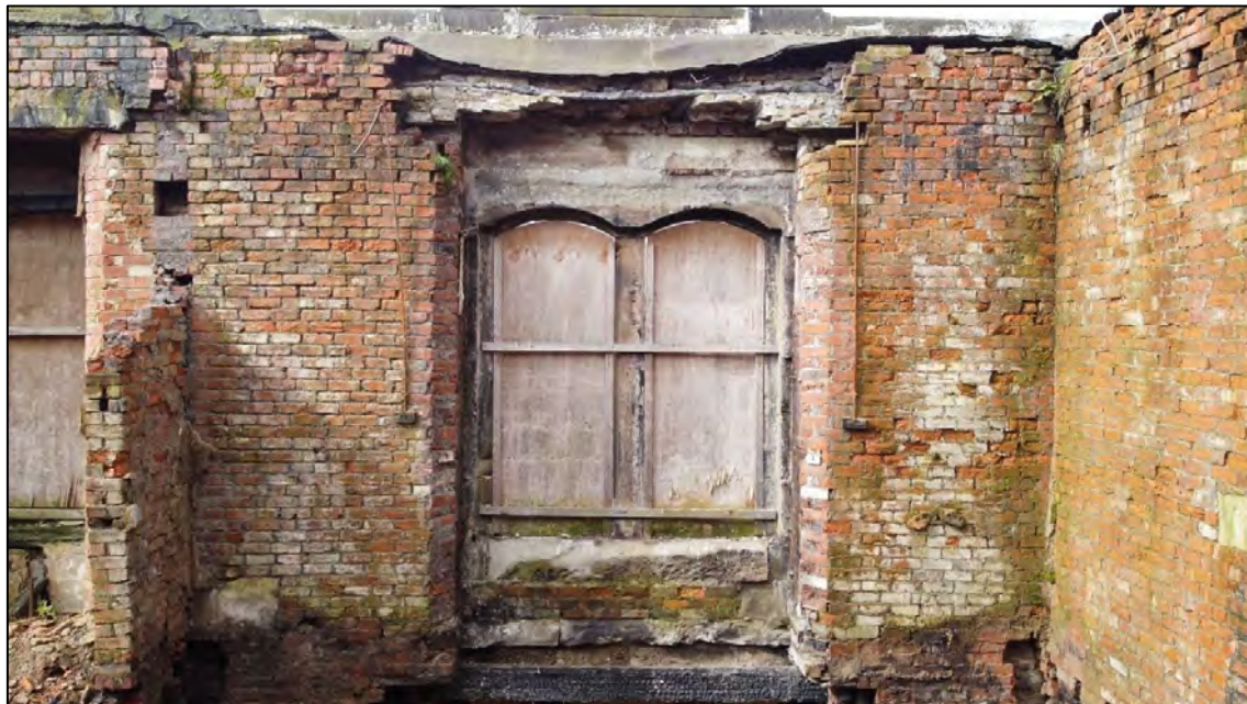
Plate 71: Internal view looking W at first floor level
