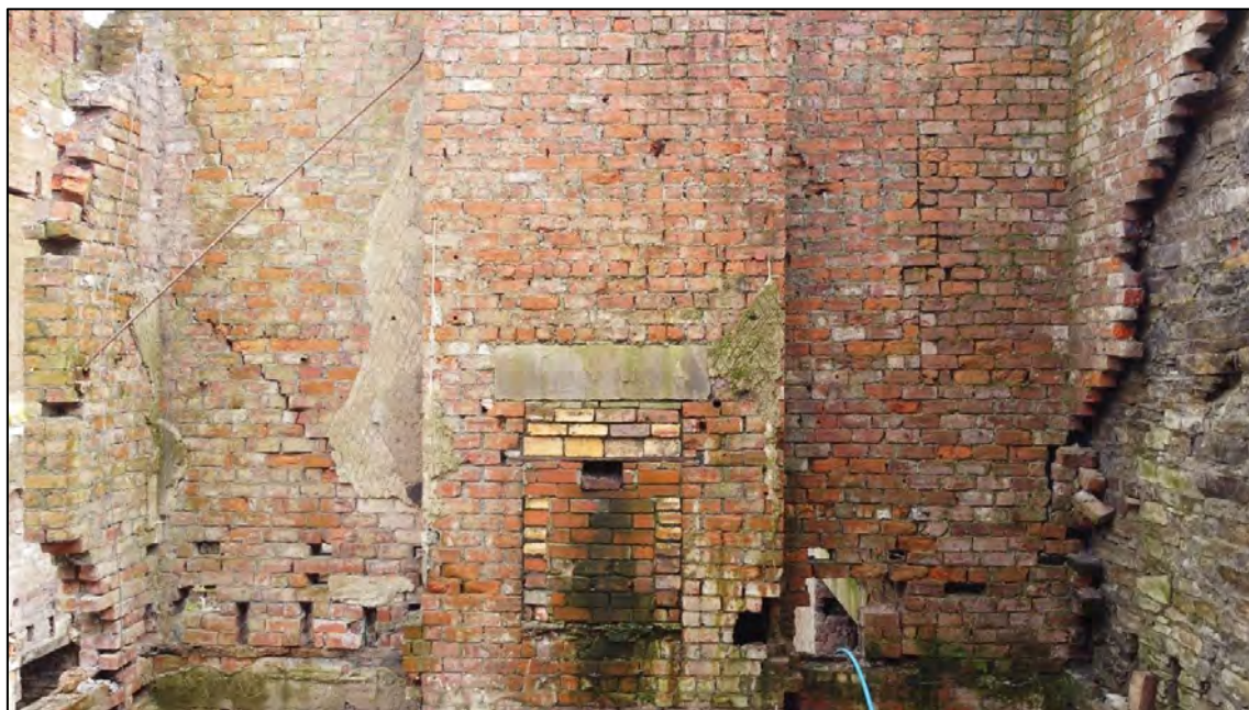
Plate 72: Internal view looking E at first floor level
