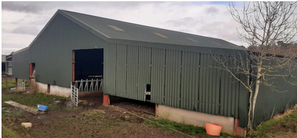
Figure 3 – Photograph of the shed from the west.
