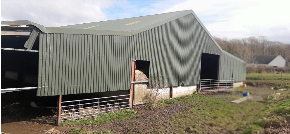
Figure 2 – Photograph of the shed from the west.
