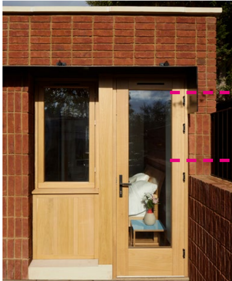
Oak doors/ windows with oak panelling and white stone base sill. Metal brise soleil
