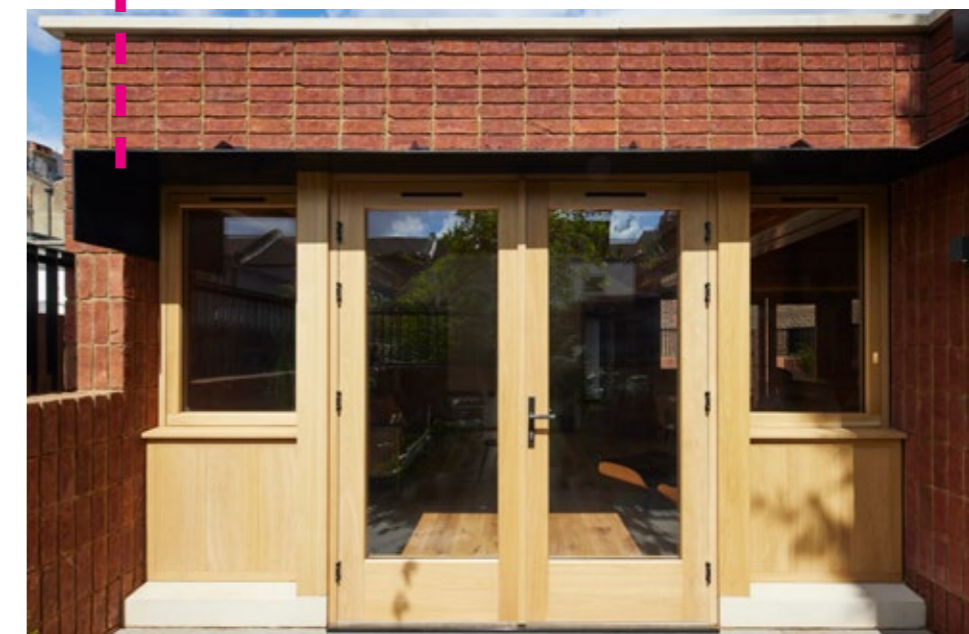
Oak doors/ windows with oak panelling and white stone base sill. Metal brise soleil
