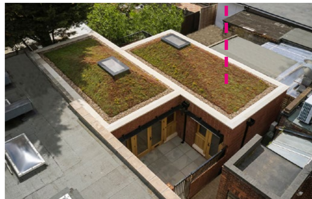
White stone parapet and extensive green roof with rooflights
