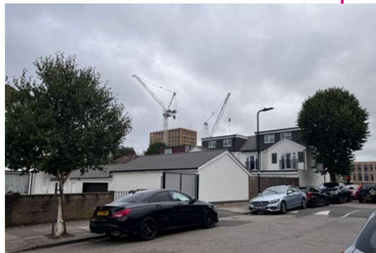
Rear of 1234 Greenford Road
