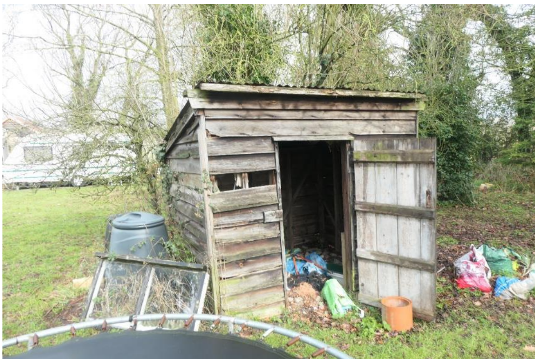
Photo 14 , south and west aspects of building four, looking northeast.
