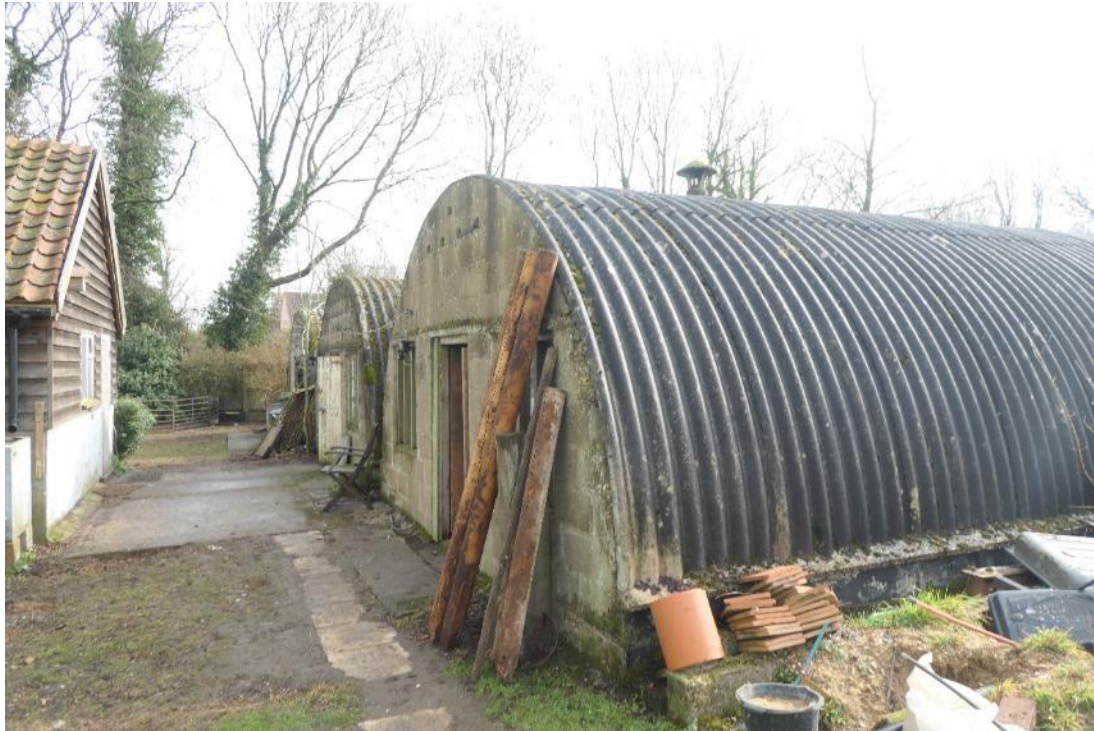
Photo 13 , north and west aspects of building three, looking southeast.
