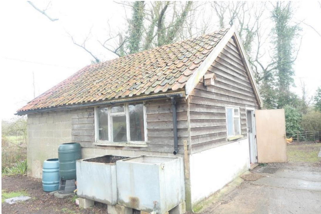
Photo 7 , south and west aspects of building one, looking northeast.
