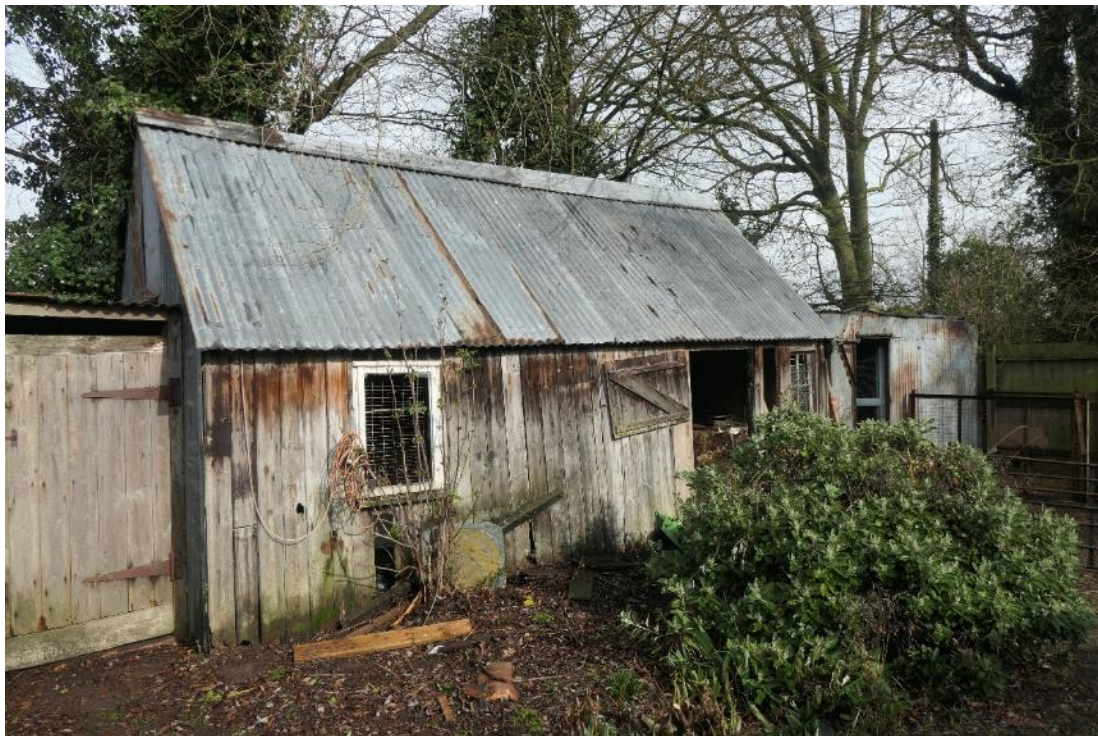
Photo 12 , south and west aspect of building two, looking northeast.
