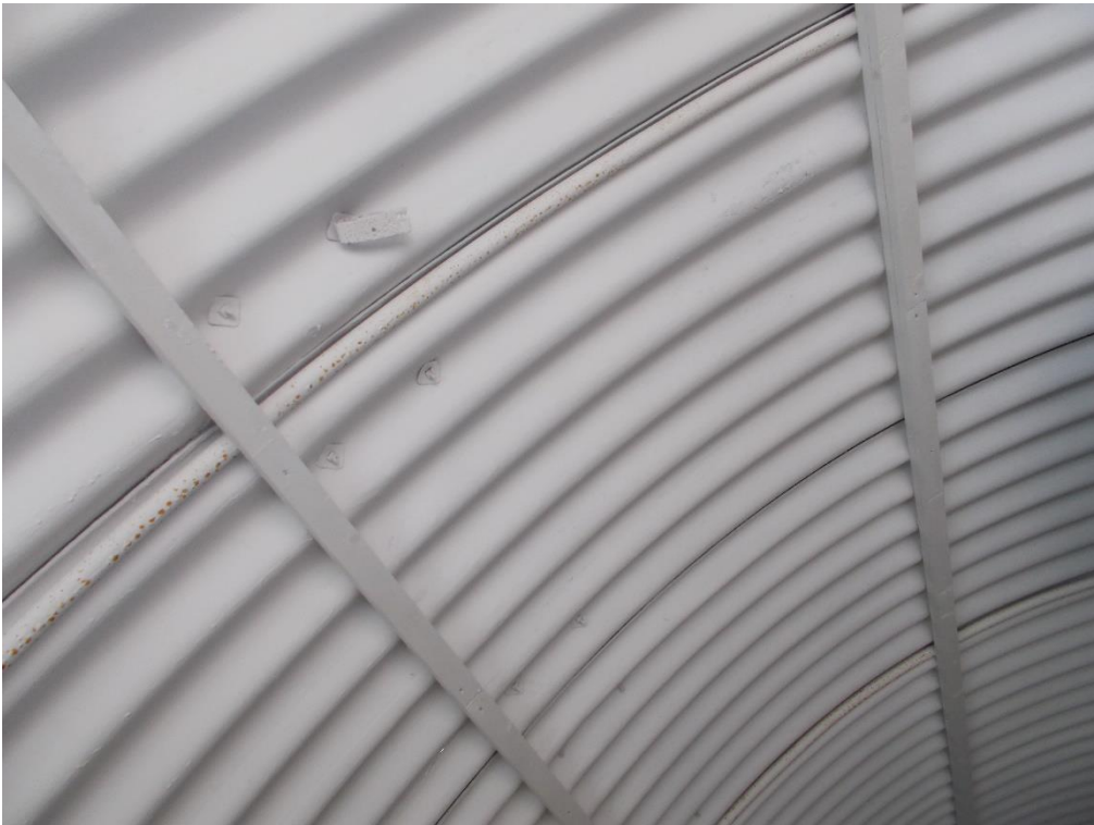
Photograph 9 – Steel rib and purlins
