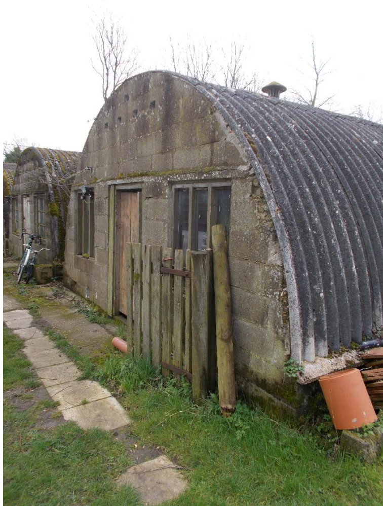
Photograph 4 – North gable ends
