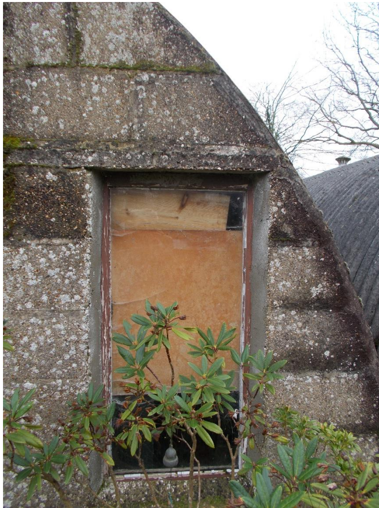
Photograph 2 – Lintel bearing
