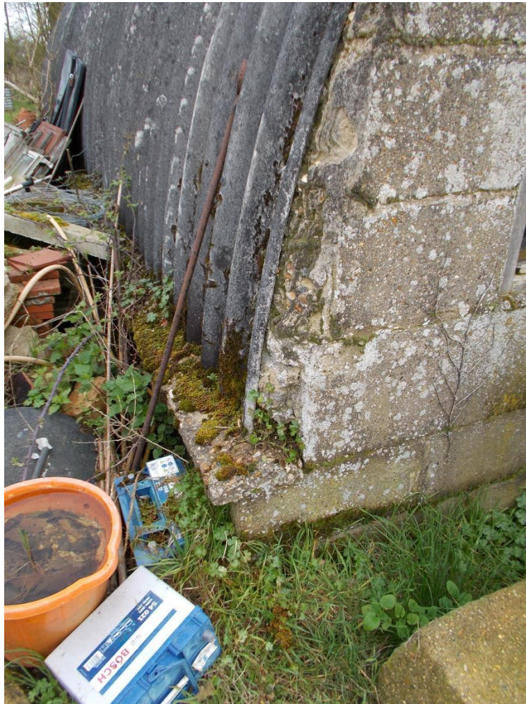
Photograph 3 – 'Springing point' concrete block plinth
