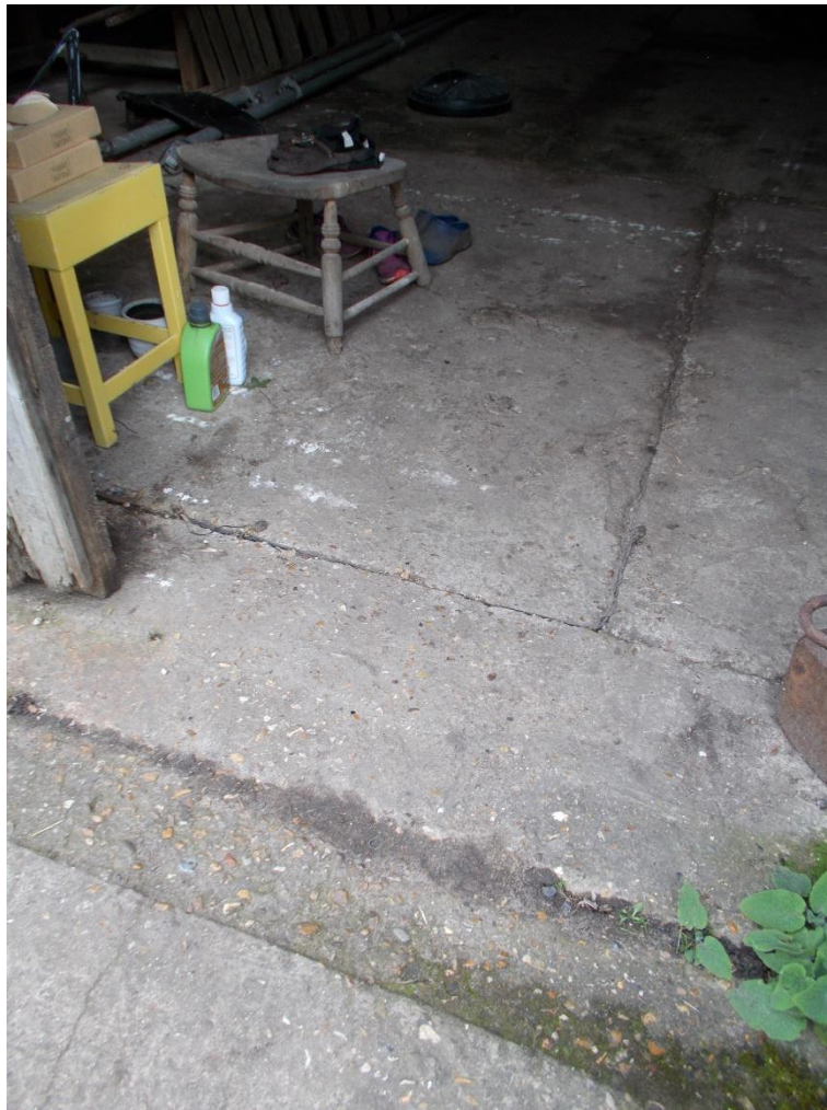
Photograph 10 – Foundation and slab details
