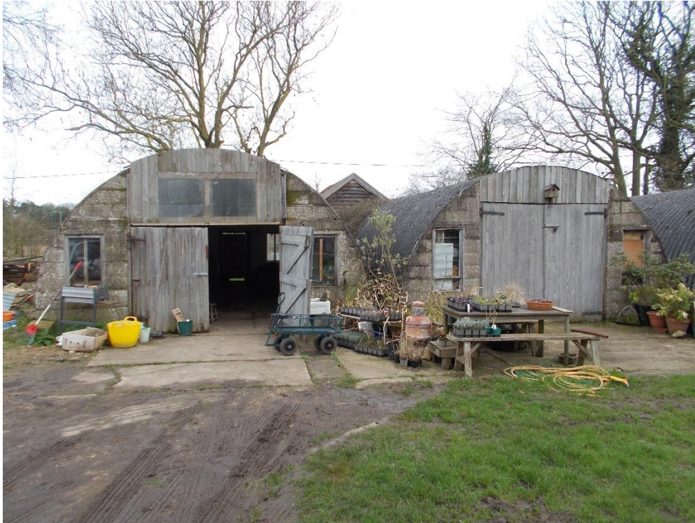
Photograph 1 – South gable ends
