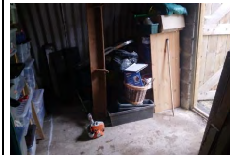
Photo 7 – eastern Nissen hut interior
