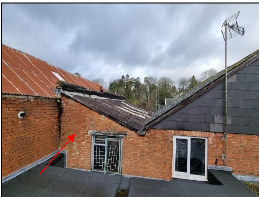
Plate 7: Rear elevation (facing north)
