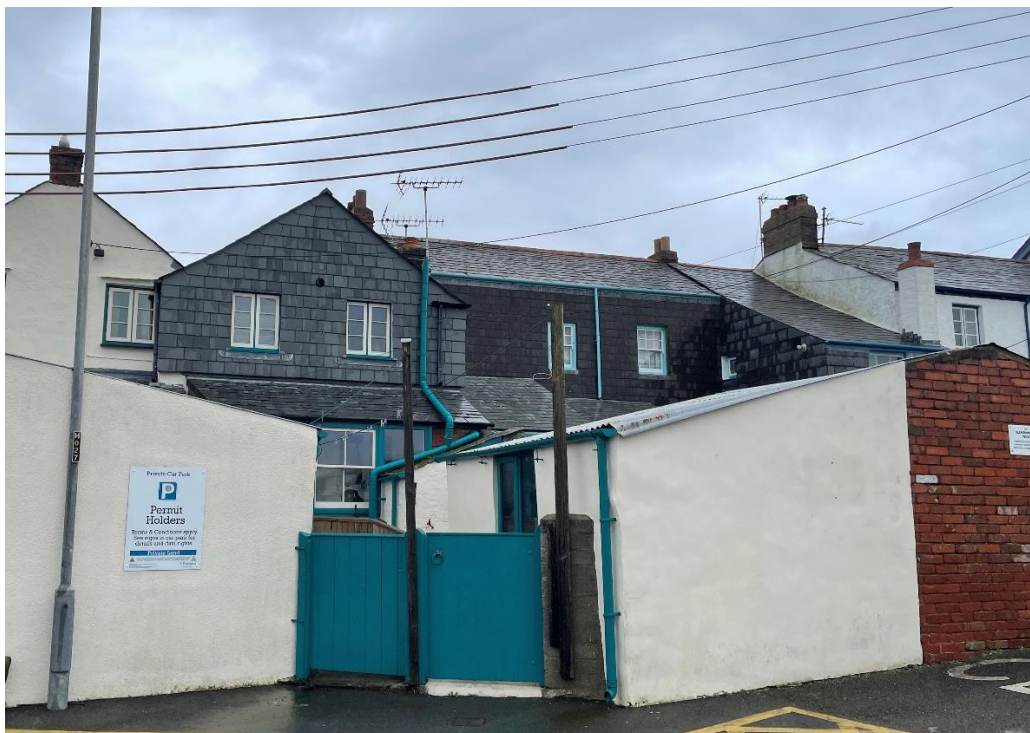
Picture above shows local buildings in Bude with slate hanging to the rear (south-west) elevations.
