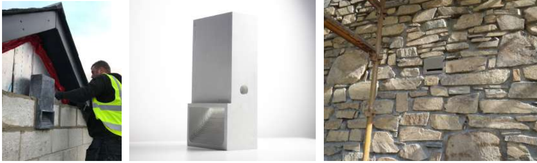
Photograph 11. 'Green and Blue' bat block and built in woodstone bat box `.
